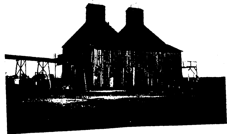
FIG. 1.—HOP OASTS. Showing cupolas, loading stage, and elevated track for the trolleys.
