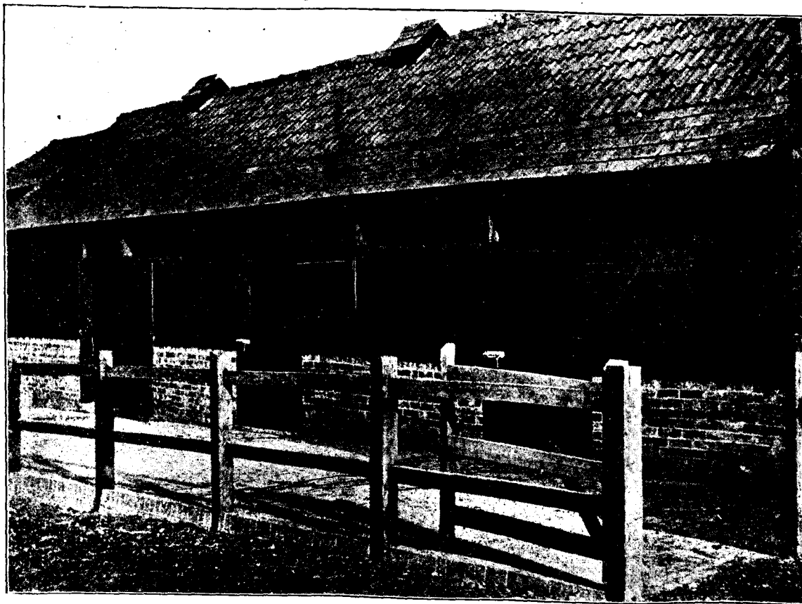
The space in front of this Cowshed for a distance of 4 yards has been railed off from yard and paved with hard bricks. Note large permanent openings for ventilation and light.
