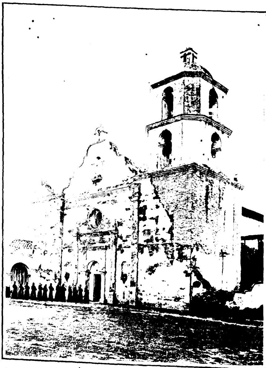
FRONT OF MISSION SAN LUIS REY, NEAR OCEANSIDE, CALIFORNIA.
