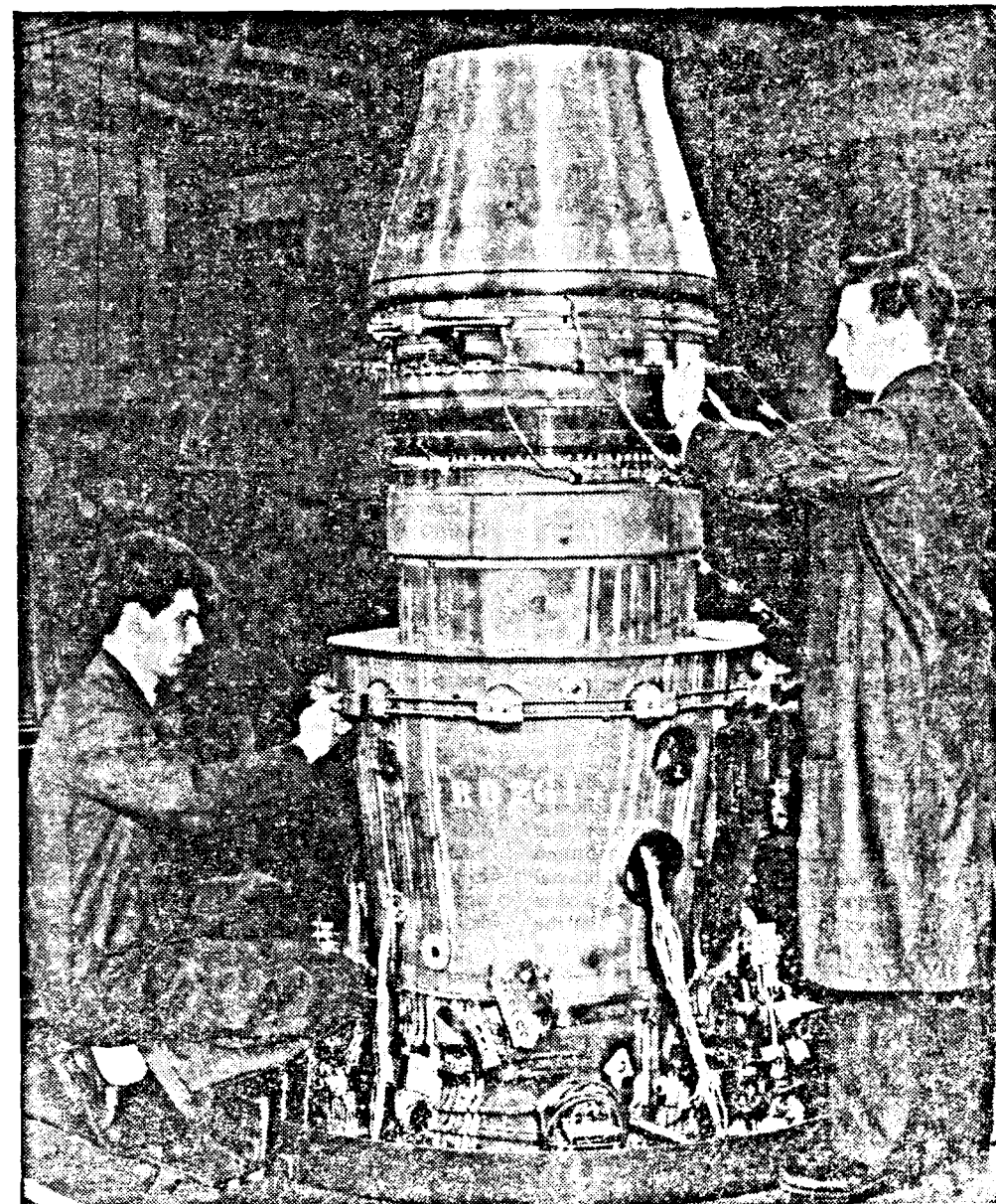
The new Spey by-pass jet engine being assembled at Derby for development testing.
