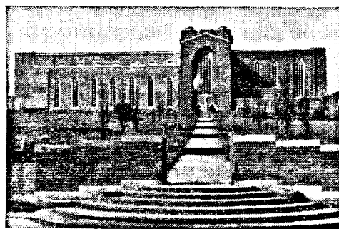
Not the ideal edifice
