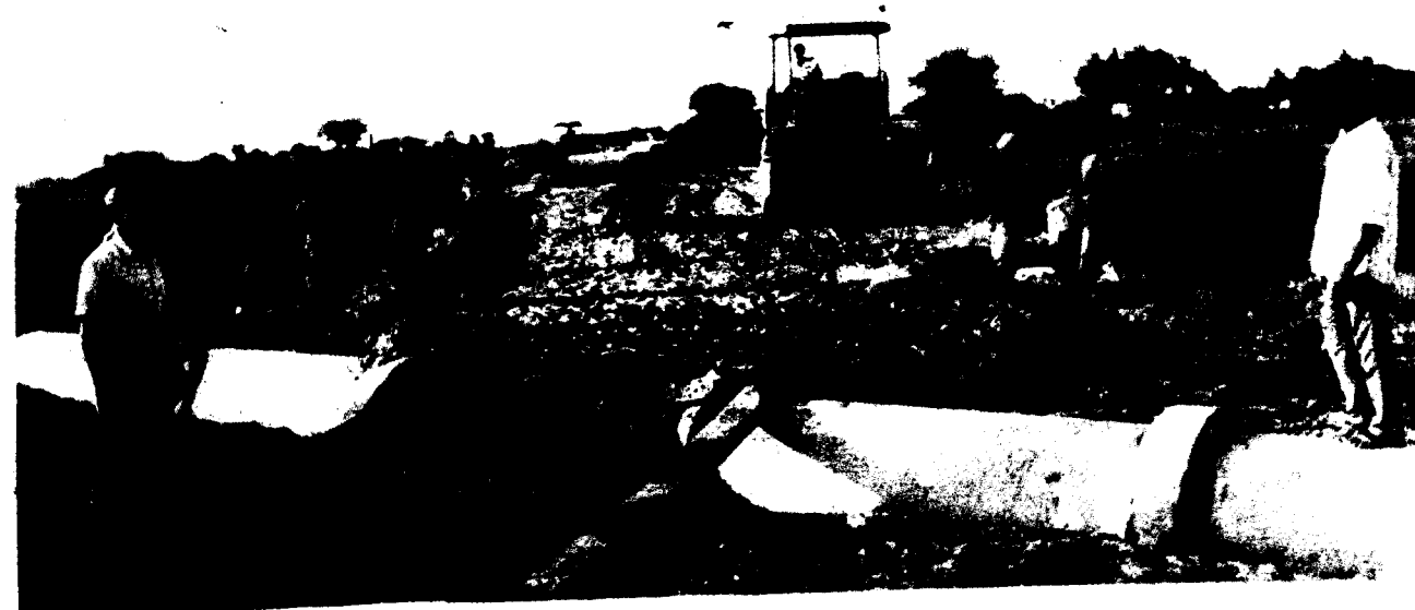
Works are on for the ring road at Thanjavur!
