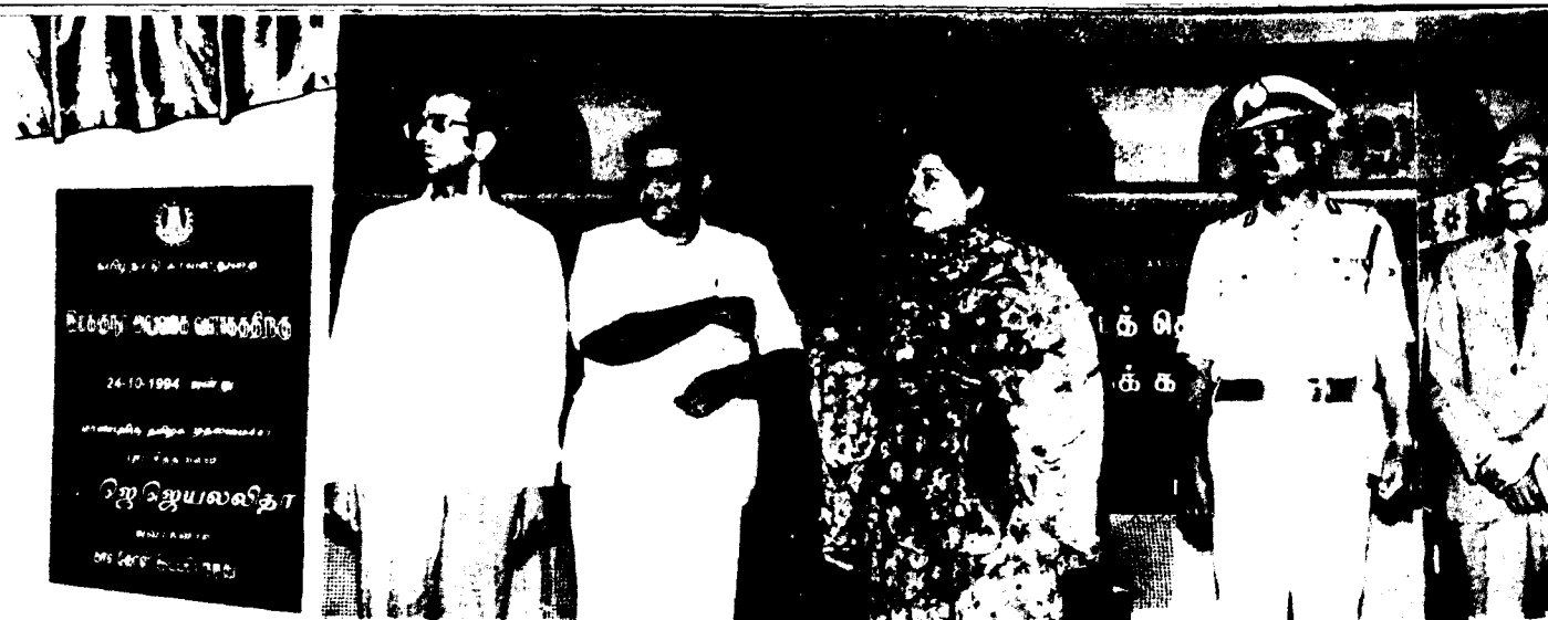
CHIEF MINISTER LAYS FOUNDATION FOR D.G.P. OFFICE COMPLEX
