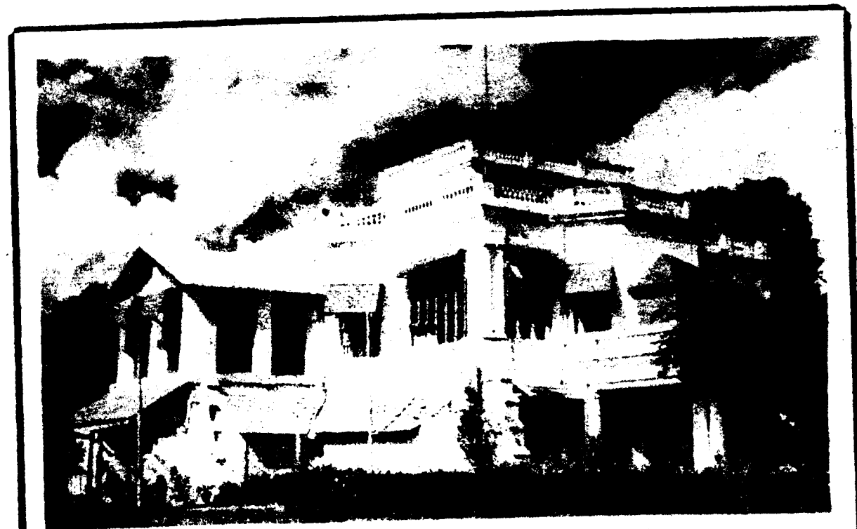
The first building that housed the All India Radio, Madras from 1938 through 1954, at 15, Marshalls Road, Egmore.
