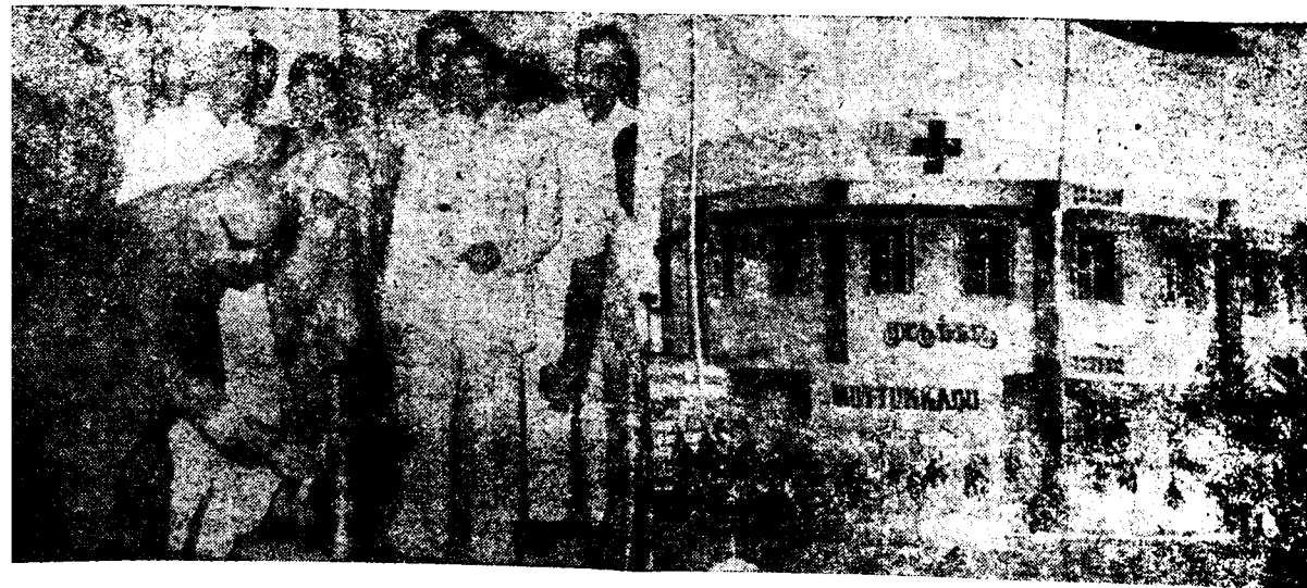
The Vice-president, Thiru M. Hidayatullah, declared opened, a cyclone shelter at Muttukadu, built by the Indian Red Cross Society in collaboration with the Government of Tamil Nadu on 19—12—'79.
