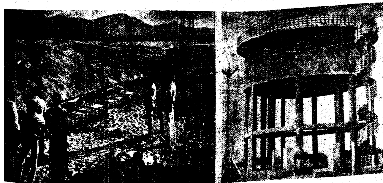
Being an essential infrastructure for promotion of industries, SIPCOT Complexes have water aplenty. Picture above shows the water-treatment plant and overhead tank at Ranipet Complex.
