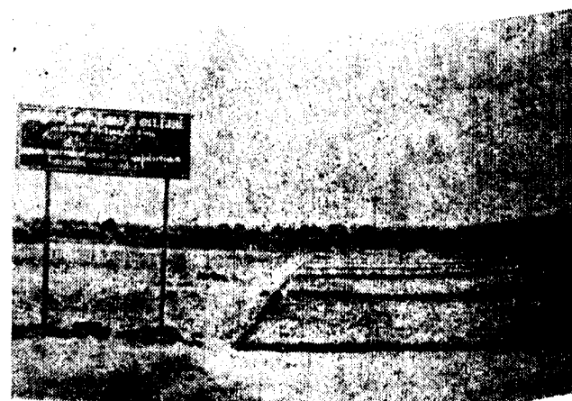
Another house-site area showing side-drains, with markings for roads at Ramanathapuram in Thanjavur dt.
