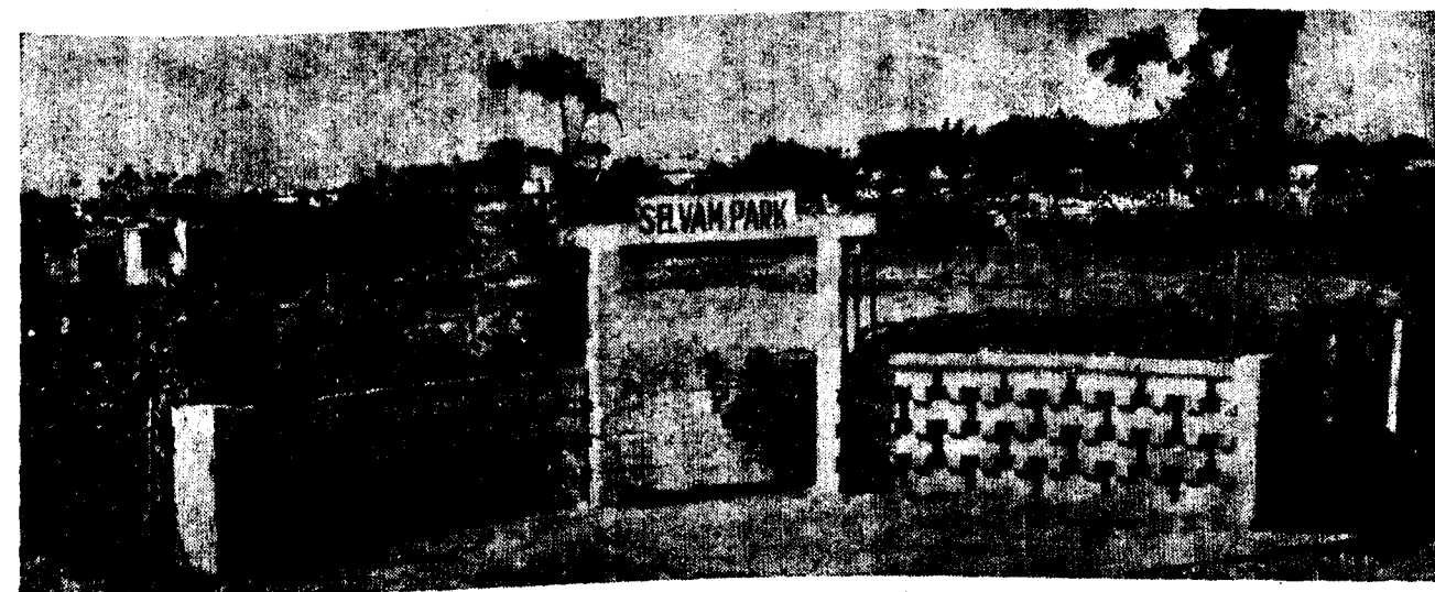
Parapet wall of Selvam Park built with celcrete
