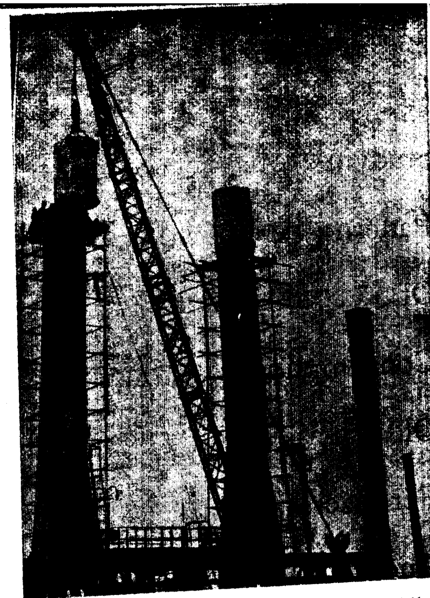
The height of the twin stacks atop the Crude furnace was extended by 3 meters each to achieve improved draft. This will facilitate efficient and clean firing at maximum crude. This height of the stack after extension is 38.9 meters from the ground level. Picture shows the progress in the erection of the stack extension piece, during September 1974. It is a huge task for conserving fuel oil in the operation of the Plant.
