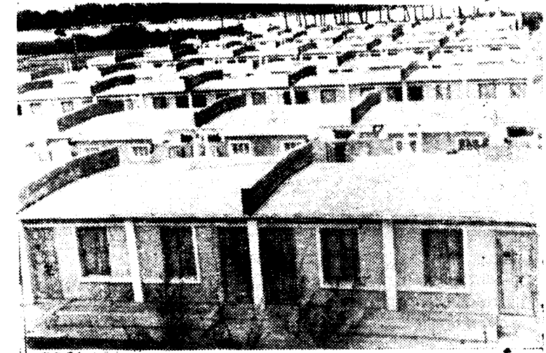
117 tenements for slum dwellers constructed at a cost of Rs. 3 lakhs at Gundusalai road, Cuddalore.
