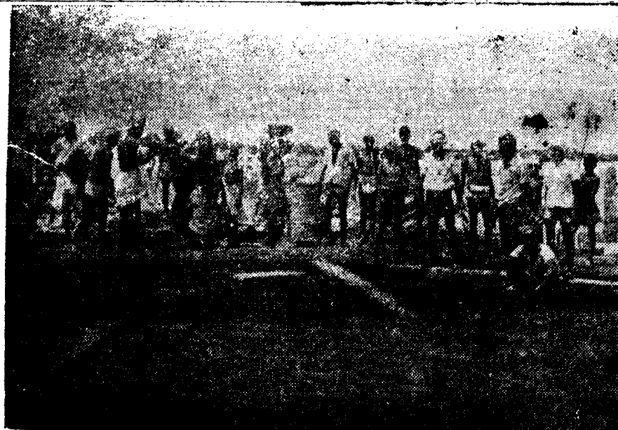
The bridge work in execution.
