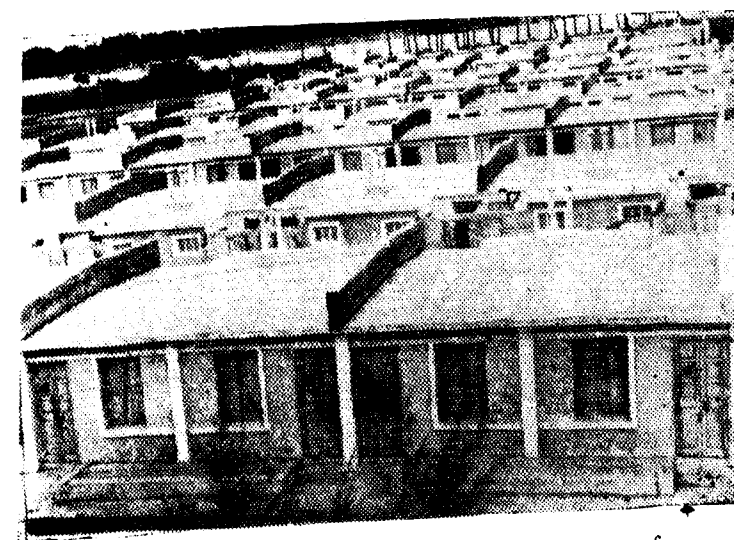
117 tenements for slum dwellers constructed at a cost of Rs. 3 lakhs at Gundusalai road, Cuddalore.
