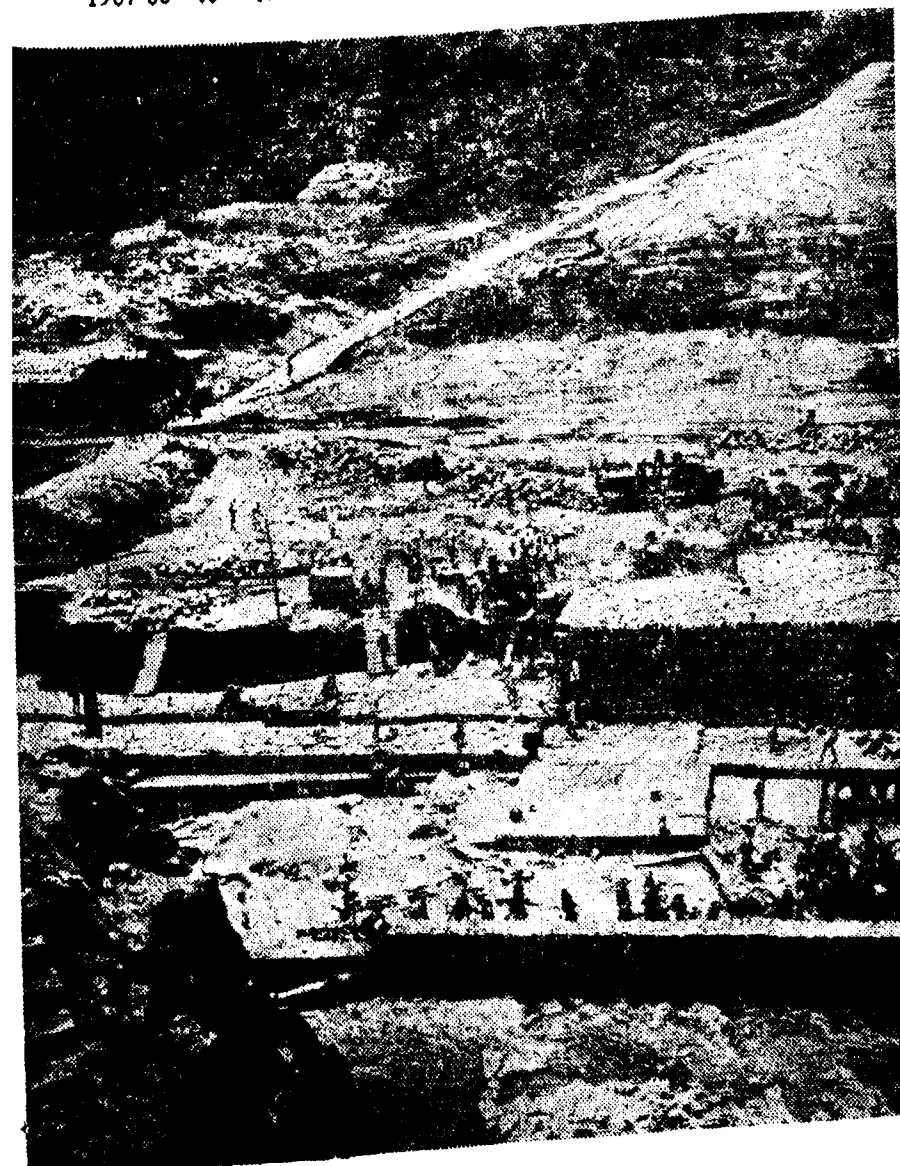
Ponnaniar Scheme under progress.
