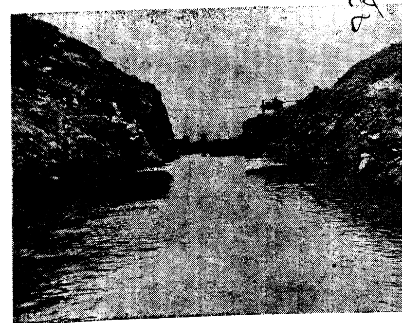
Original course of the river before construction.
