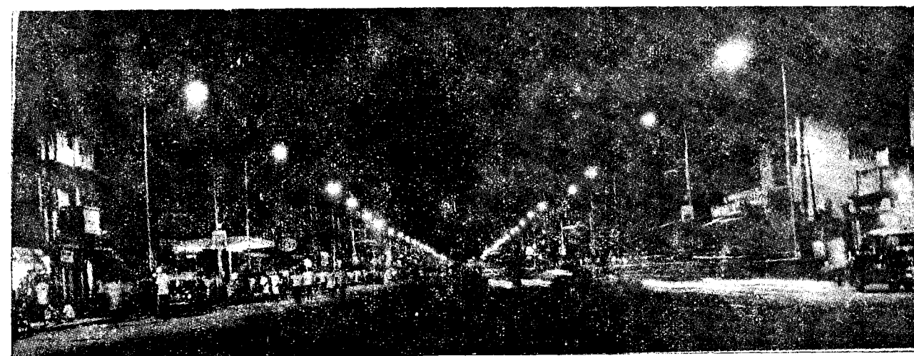
The Mercury discharge lamps which light up main roads.
