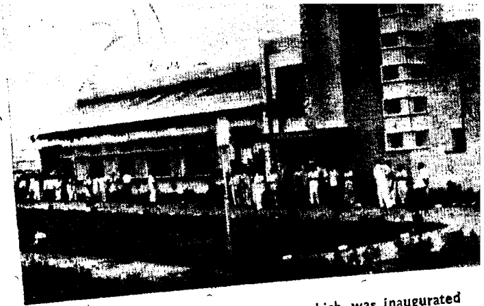
A view of the General Purpose Workshop which was inaugurated by the Chief Minister of Madras on 11th October 1965.
