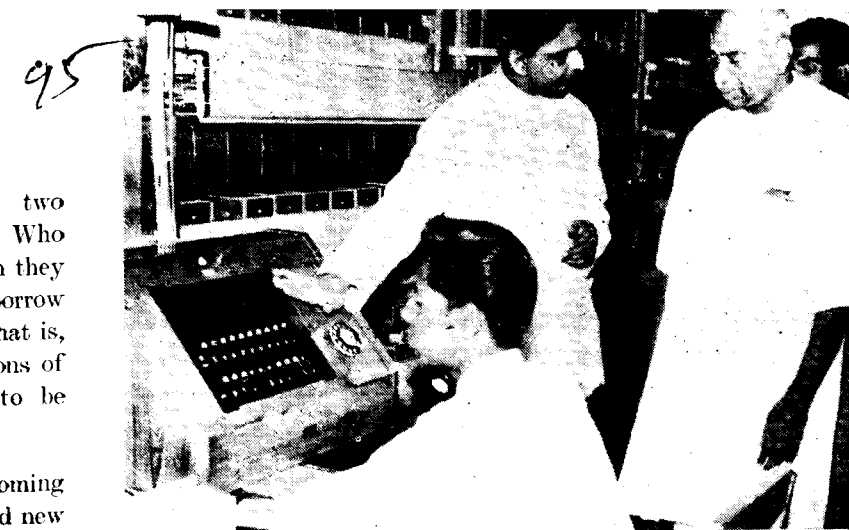
Equipment at the St. Thomas Mount Automatic Telephone Exchange being explained to the Chief Minister.
