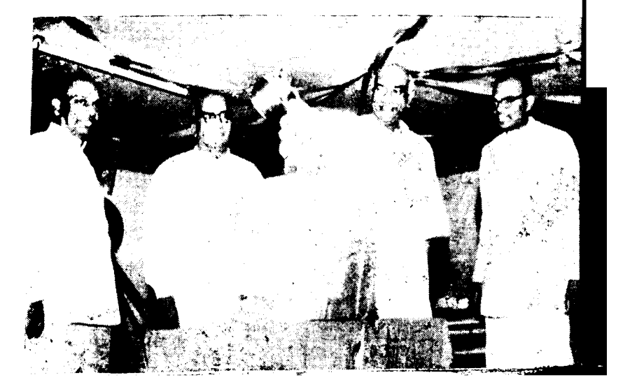
Chief Minister Kamaraj, recently laid the foundation stone for the Government Public Works Workshops and Store Workers' Colony at Tondiarpet, Public Works Minister Ramaiah presiding.
