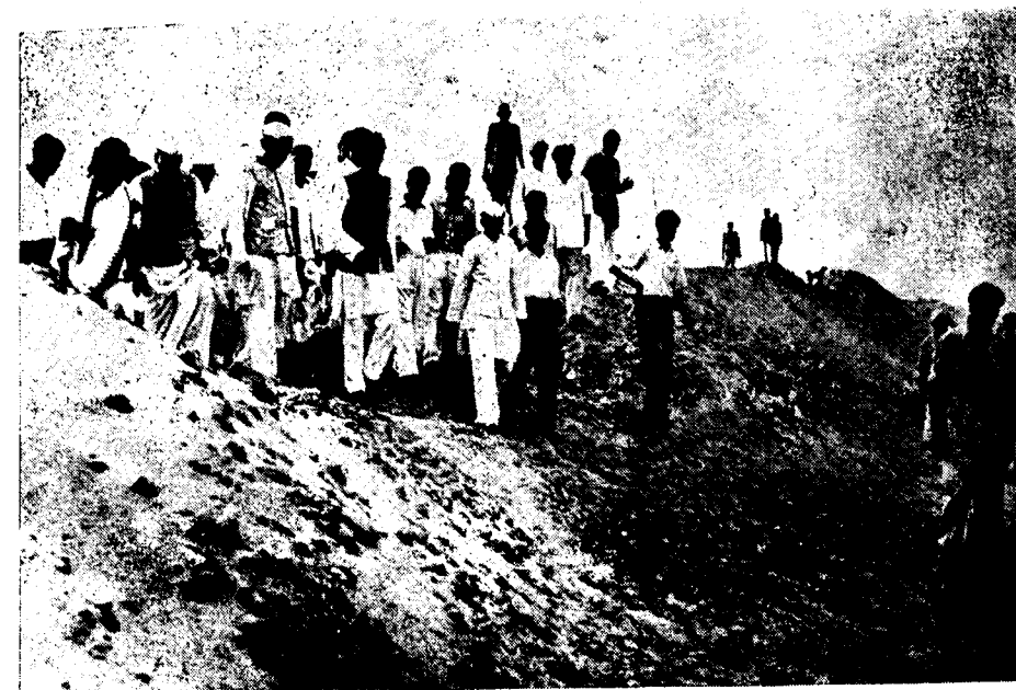
Shri Gulzarilal Nanda, Union Minister for Planning, visited the site of the Shahdara Bund on June 21 when he saw a mile-long embankment constructed by members of the Students' Camp conducted by the Delhi State Bharath Sevak Samaj.
