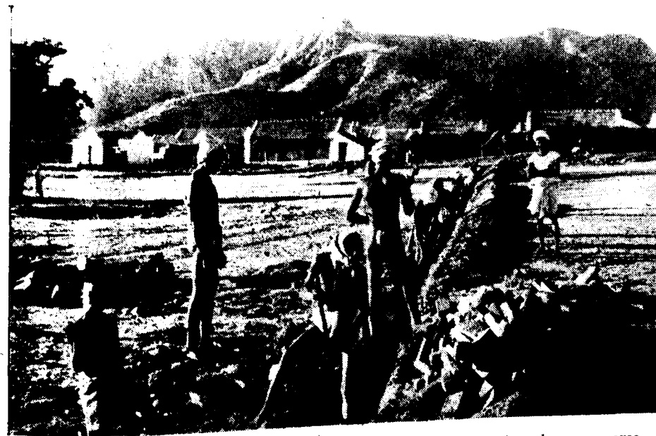
Villagers laying pipe-lines for drainage under the Local Development works programme.
