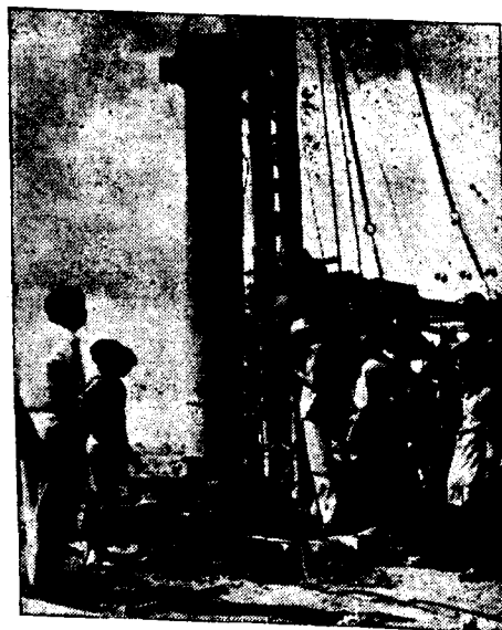
After drilling, the holes had to be protected by steel-casing and prepared for pumping.
