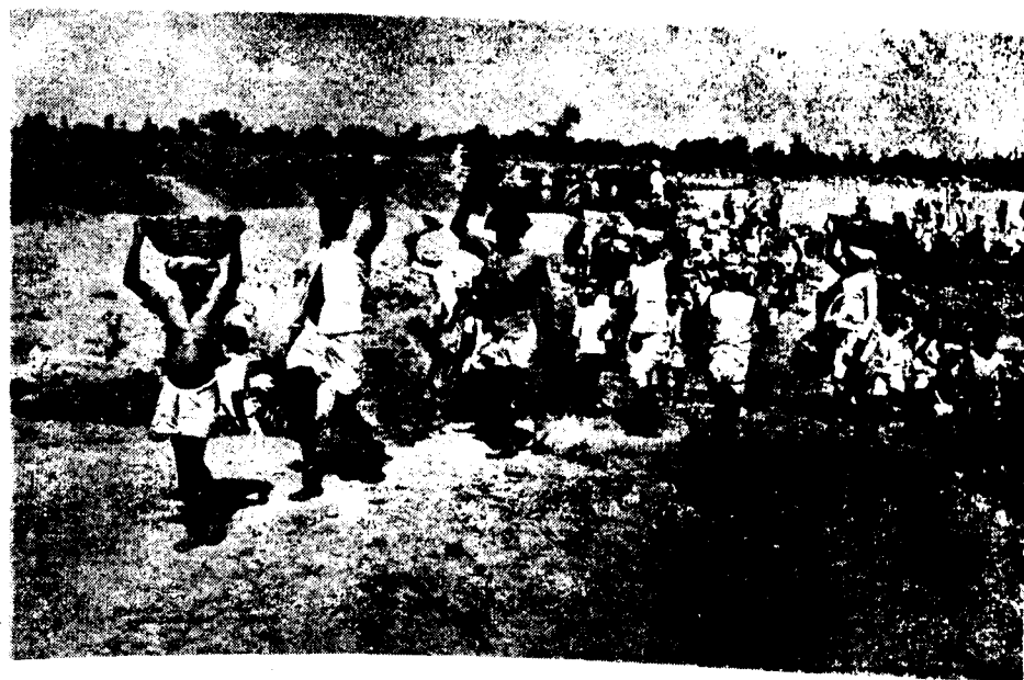
Villagers offering "Shramadan" in a village for the construction of an embankment. The Second Plan provides large opportunities for co-operative action.
