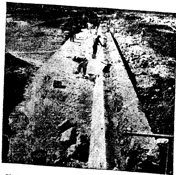
CLOSE-UP OF THE DAM WALL: The 150 feet dam wall at Palekythro, near Kythrea, part of a scheme which the Cyprus Government is carrying out to combat the drought damage.
