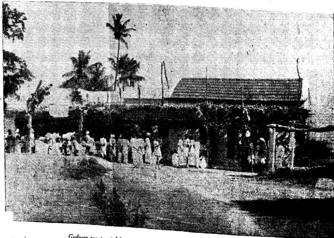
Godown constructed by the Baireddipalle Co-operative Society (Chittoor district).
