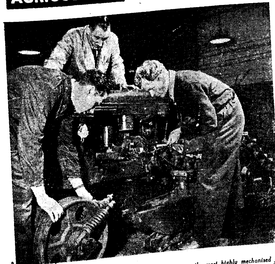
FARM MECHANIC TRAINEE LEARNS HOW: Farm students at the tractor repair section of the United Kingdom Government Training College at Letchworth, in the county of Hertfordshire, being instructed in the assembling of a track tensioner wheel of a track laying tractor.
