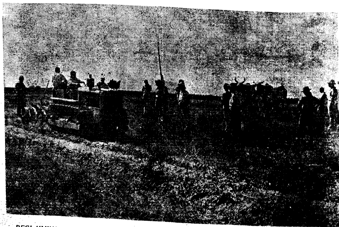
RECLAIMING WASTE LAND: Land Army workers reclaiming 43-acre sandy, weed-infested plot in the village Qomurudin Nagar. Tractors helped in it.
