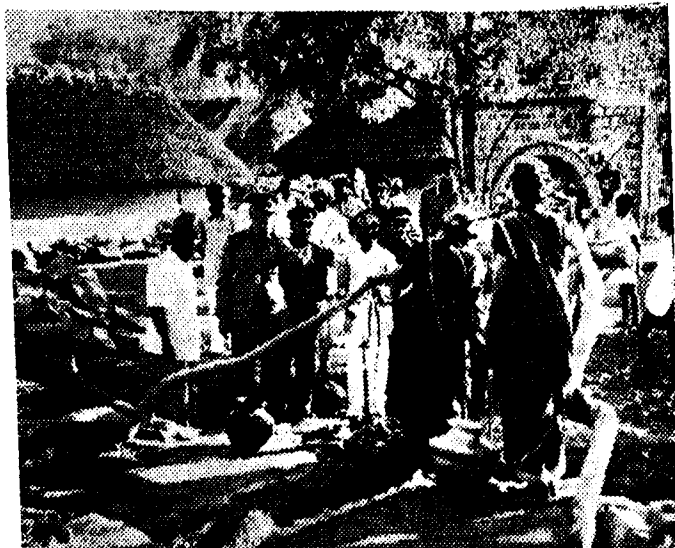
WELL INSPECTION: General Cariappa inspecting a dried up well along with the local officials, in the distressed areas.
