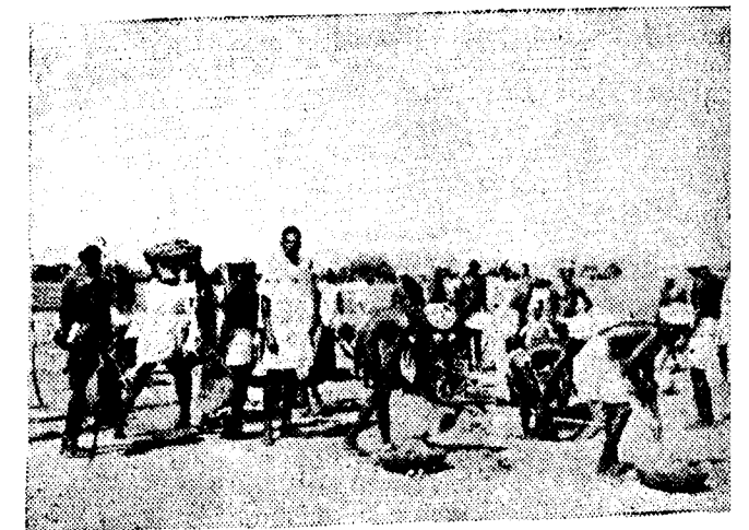
YOUNG AND OLD took part in the construction, with only a short midday break. Crowbar, spade and basket were used to good purpose.
