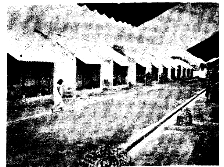
A neat array of houses in a Harijan colony
