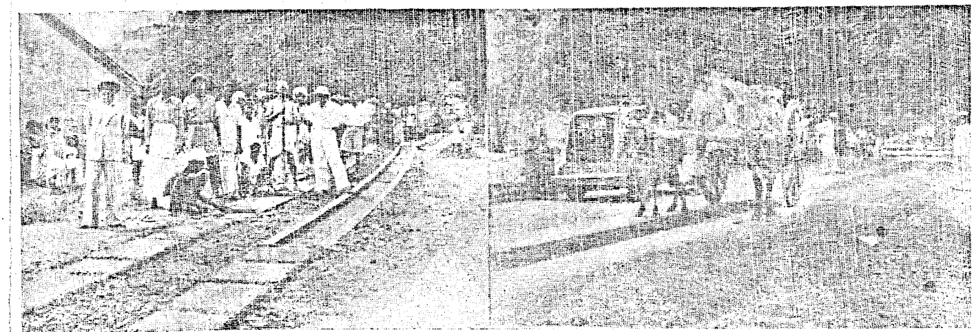
Creeways (Cement Concrete Tracks) on Kancheepuram-Wandiwash Road: (left) work in progress and (right) the finished work
