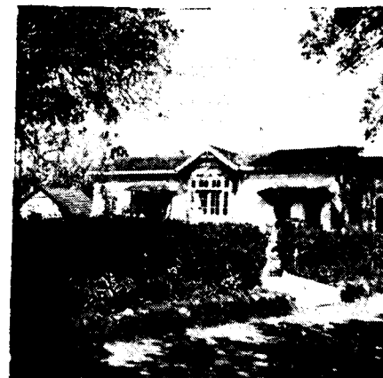
Stores and Admn. Block.
