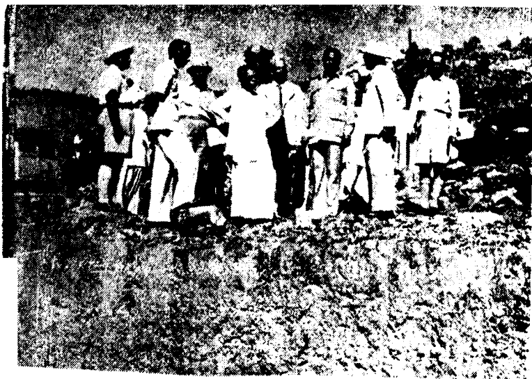
The Hon'ble Ministers and officials of the Public Works Departments of Madras and Orissa visit the project sites and review the progress made
