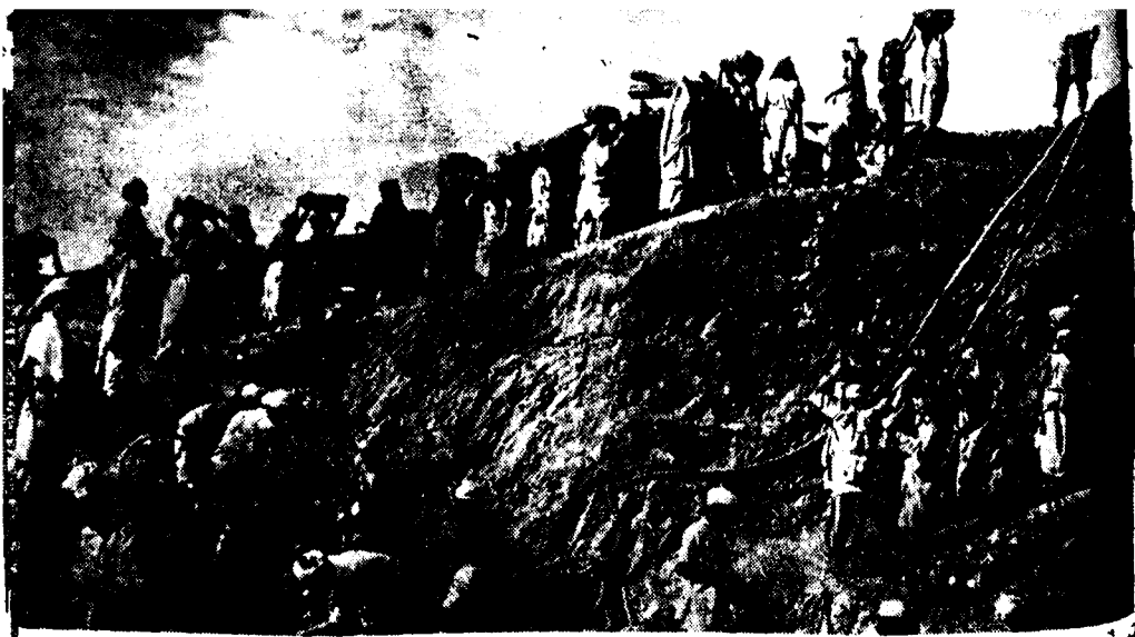
Man power to harness Nature: Work proceeding ahead at the Tungabhadra Project
