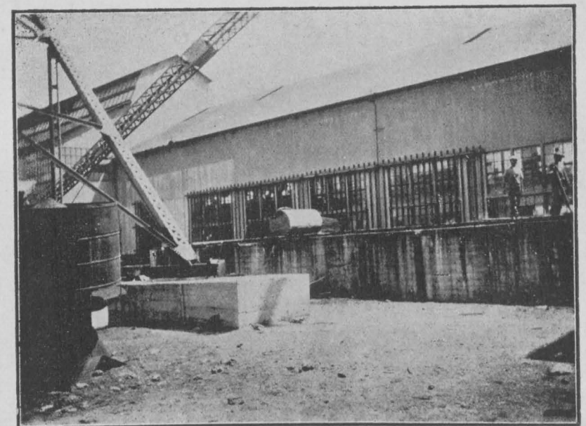
6. CONCRETE BOILING VATS SHOWING A LOG READY TO BE PUT IN BEFORE BEING CUT BY THE ROTARY PROCESS.
