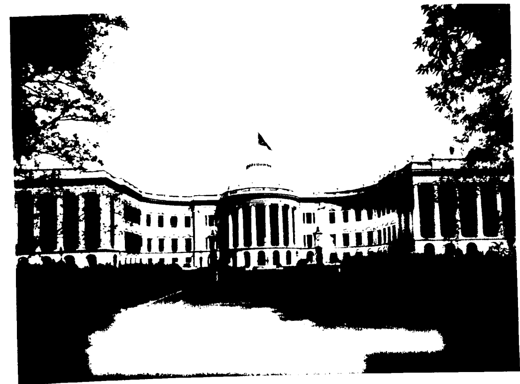
GOVERNMENT HOUSE, SOUTH FRONT (1903)
