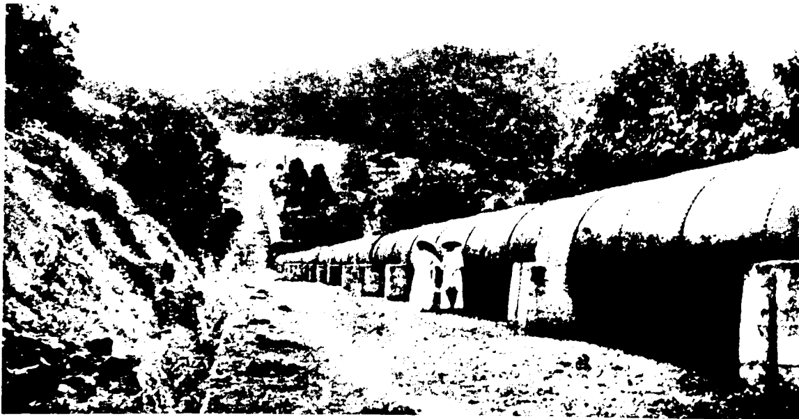
Tata Hydro Electric Works; 82-inch pipe near Forebay.
