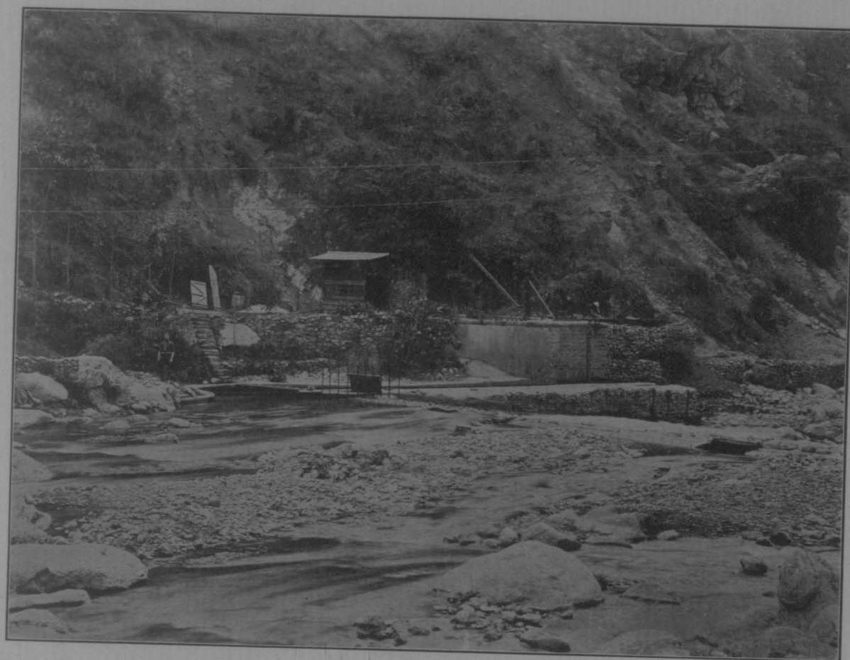
Simla Hydro Electric Works; The Head Works.
