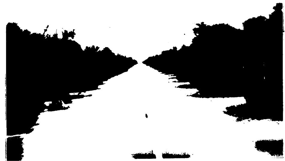
(a) Open Masonry Furrow Distributory, supplying irrigating furrows through small furrow-gates in sides. Irrigating on left; on right, harrowed after irrigation.
