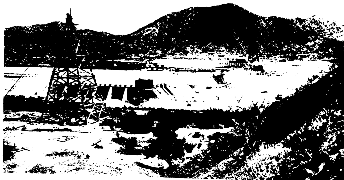
c. Granite Reef Weir during construction from right bank.
