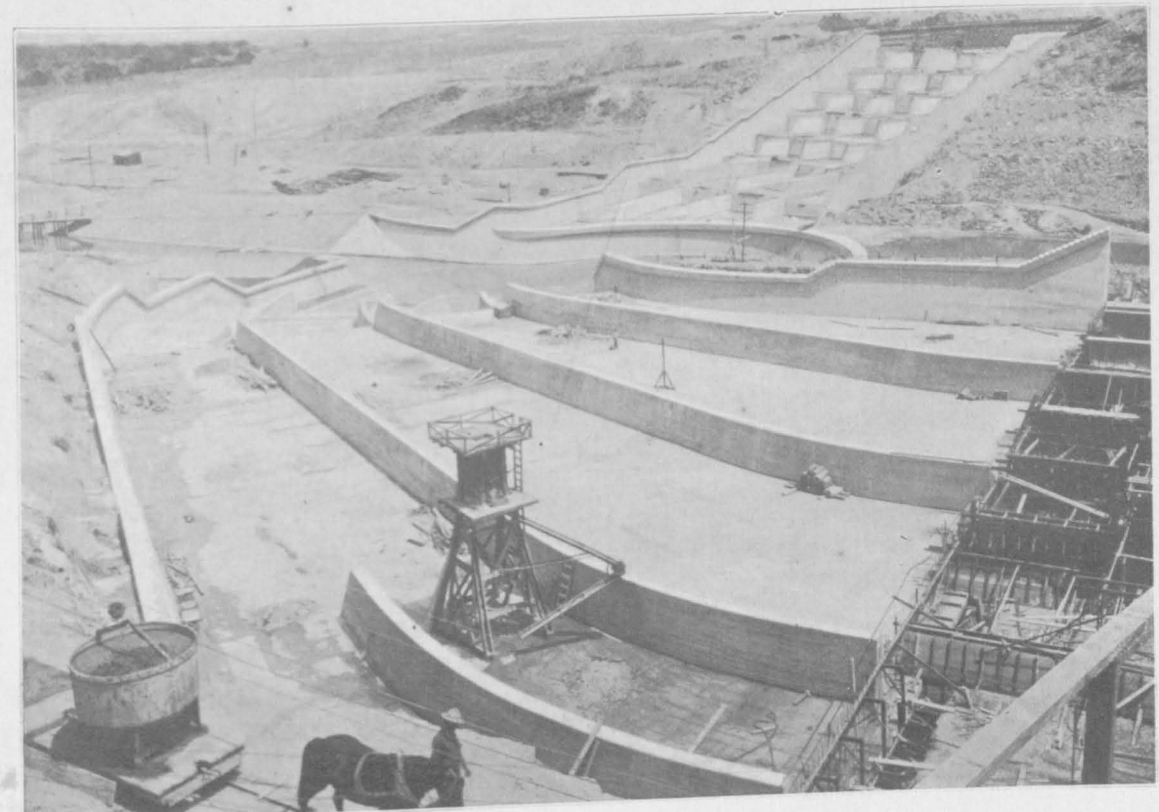
(a) Lower parts of both Spillways. Note concrete bucket on horse-truck and distributing hopper on movable tower.
