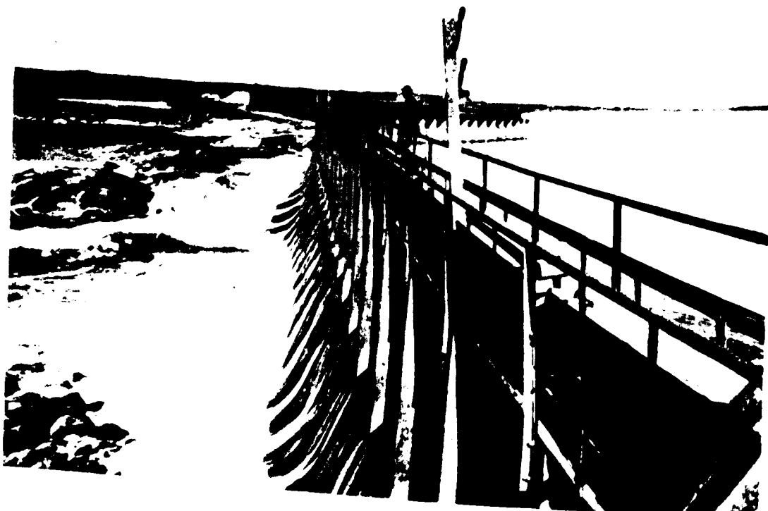
d. Part of Overflow Weir.
