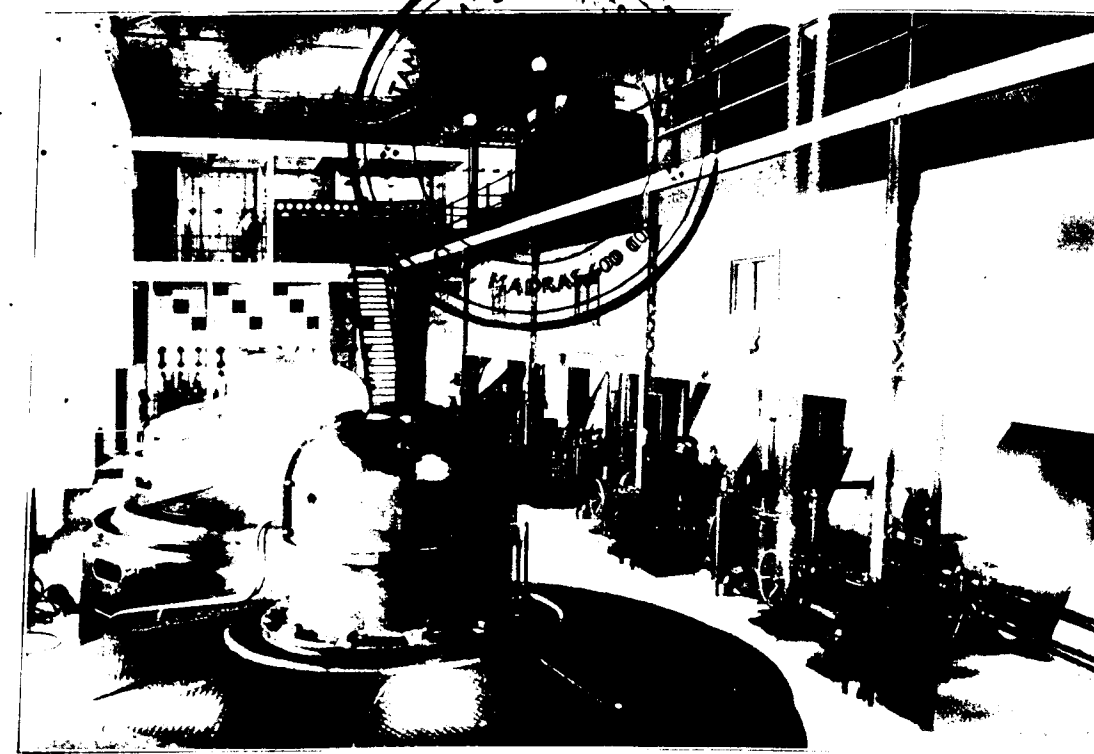
(b) Inside of Power-house.
