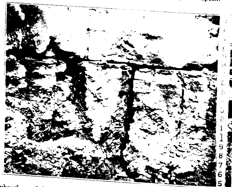
(c) Typical Subsurface of Cracked Clay Material. The bottom of the rod is 5.3 ft. below the surface. From paper by H. T. Cory, Vol. 38-39, Proc. Am. Soc. C.E.
