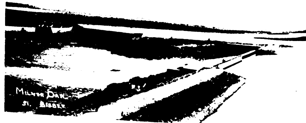
(b) Weir from left bank, near entrance to South-side Canal. North-side Canal Wall visible across river on l
