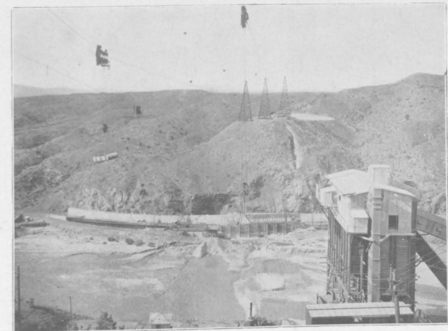
(a) From left bank. Diversion-flume on right of river. Concrete-mixing plant in foreground.
