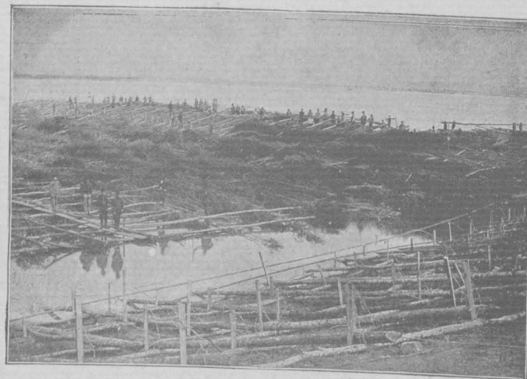
Woven Mattress under Construction.
