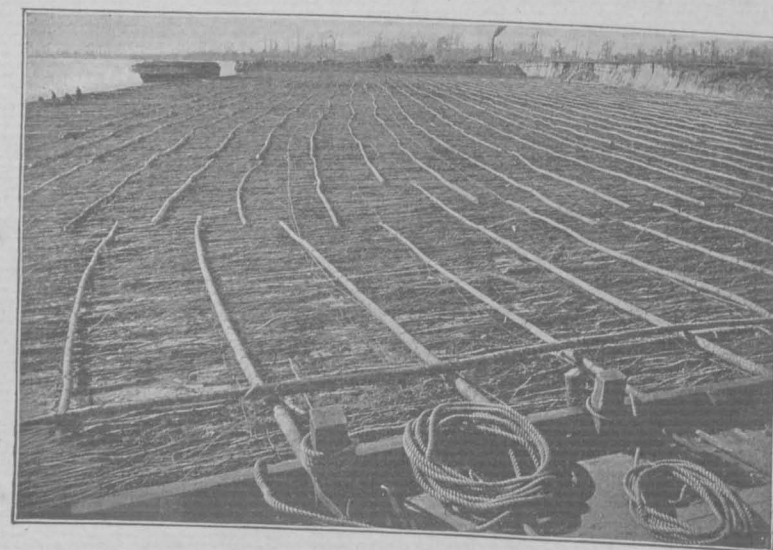
Fascine Mattress, Completed. 300×1125 feet.
