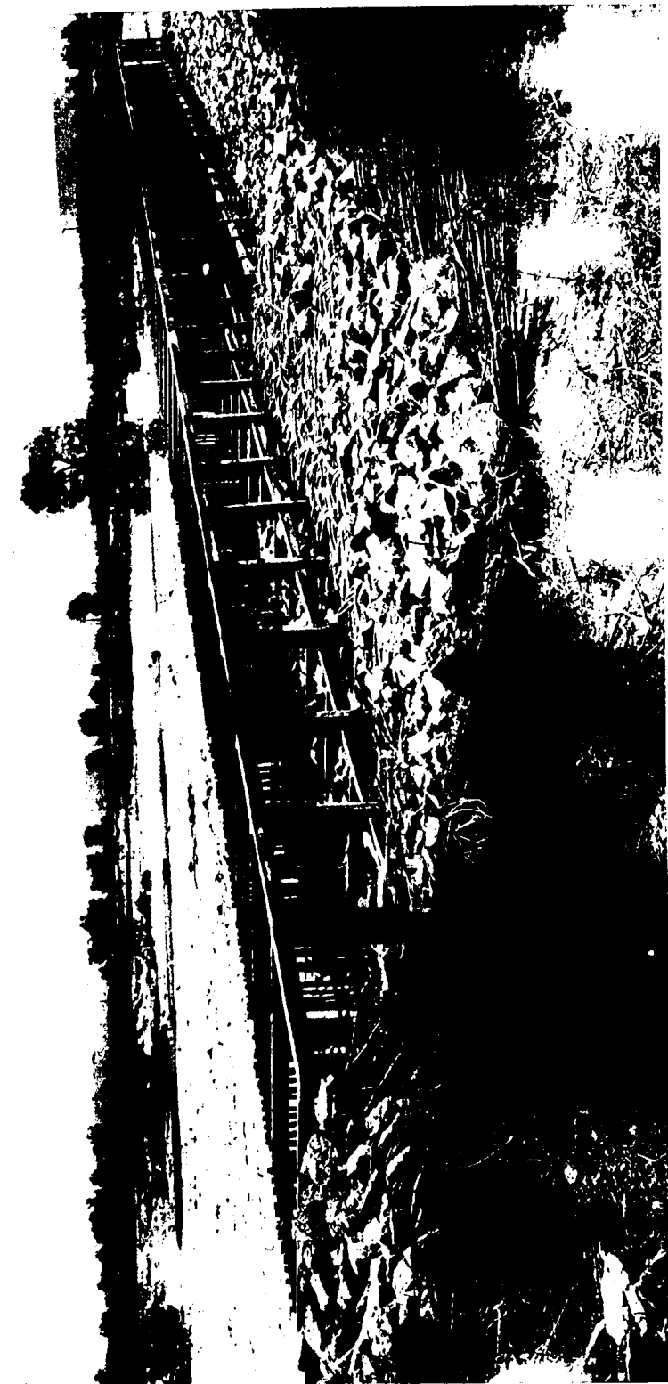
FIG. 90.—Permeable Dike with Pole Screen, and Concrete Piles and Braces. Constructed in 1910 on the Republican River, at Fort Riley, Kansas.
