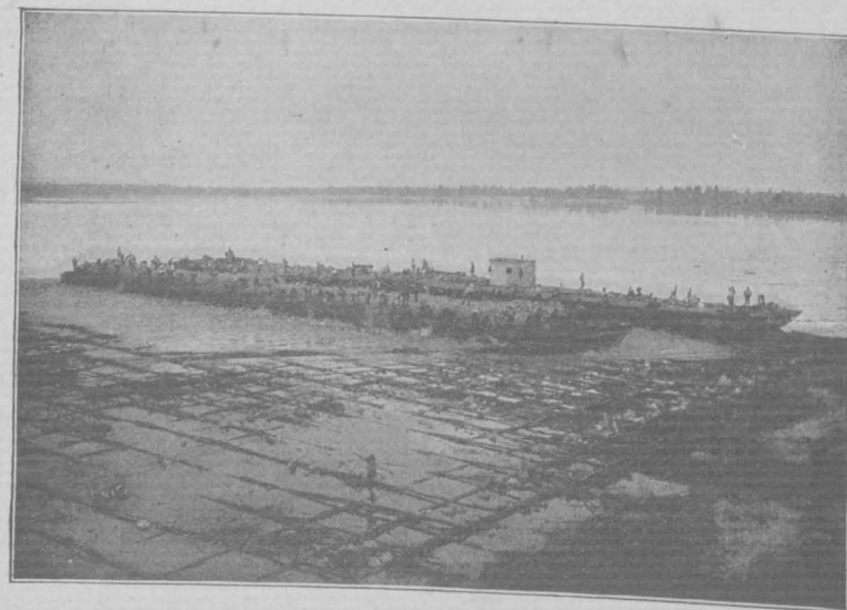
Woven Mattress just Beginning to Sink.
