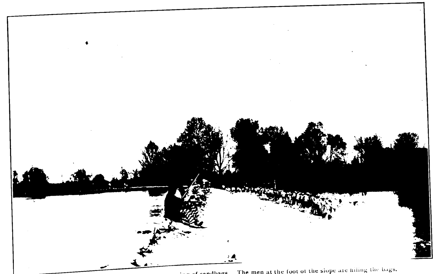
A sand-boil on the land slope of a levee, protected with sandbags. Note also the layers of sandbags used to stop the sloughing of the slope and the seepage water beyond.
