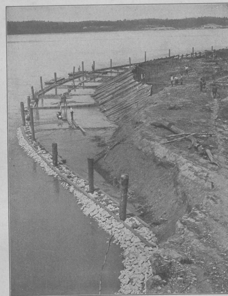
FIG. 115.—Bank-head near Chamois, Mo., Nearing Completion. Looking Downstream.
