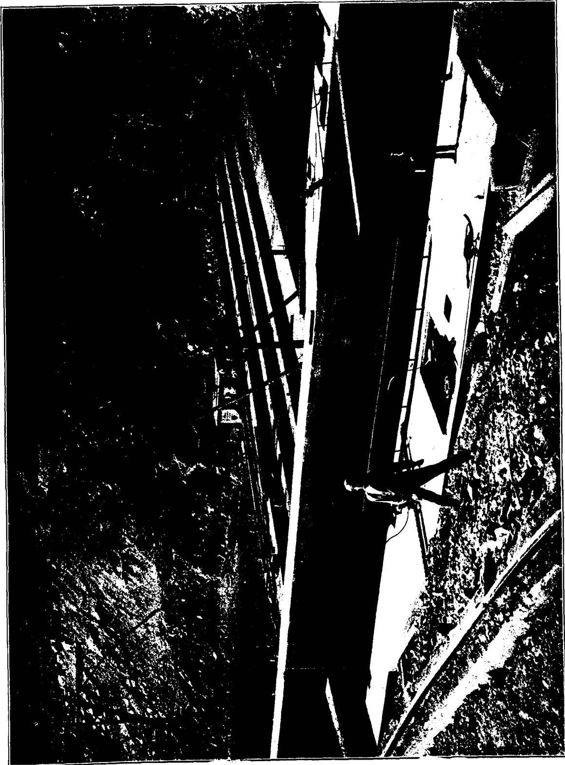
GENERAL VIEW OF DAM No. 7, KENTUCKY RIVER, KENTUCKY, U. S. A., DURING CONSTRUCTION. The dam is of the step type and built of timber cribs filled with riprap. The length is 350 feet, with a base of 60 feet. The lift is 15½ feet. The dam was completed in 1897.
