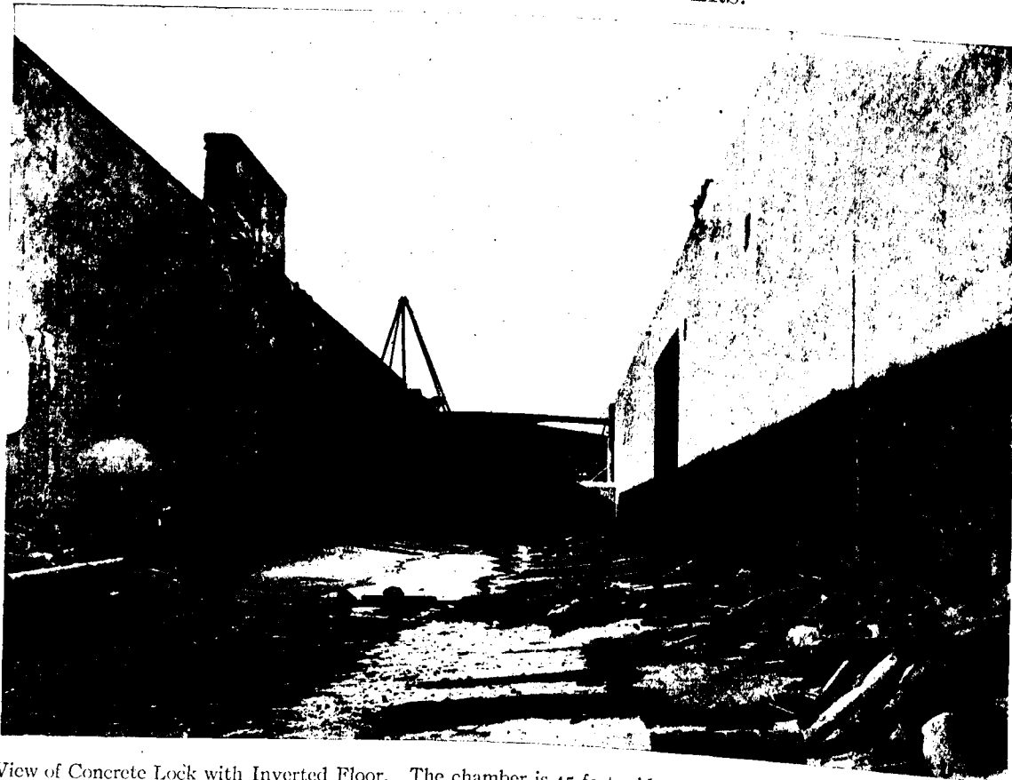
View of Concrete Lock with Inverted Floor. The chamber is 45 feet wide with a depth on the upper miter-sill of 16 feet and a lift of 15 feet. The floor is 3 feet thick, with piles embedded in the concrete. (Cranesville, Mohawk River, N. Y., 1909.)
