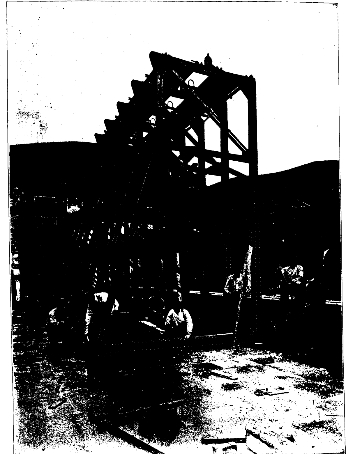
VIEW SHOWING TRESTLES FOR BOULÉ GATES AT THE LIBSCHITZ DAM, BOHEMIA, TAKEN DURING CONSTRUCTION.
