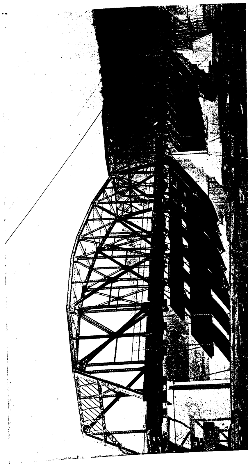
Dam at Crane's Village during Erection of Steel Work. This dam has one center span of 180 feet clear and two side spans each of 150 feet clear. Depth on sill, 20 feet; normal lift, 15 feet; uprights, 15 foot centers; gates 29 feet 8 inches long, in two tiers. All masonry is of concrete.
