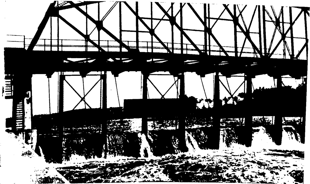
Regulation by Overflow and by Maneuvers of Gates, showing one of the upper tiers of gates raised to assist in passing a small flood.
