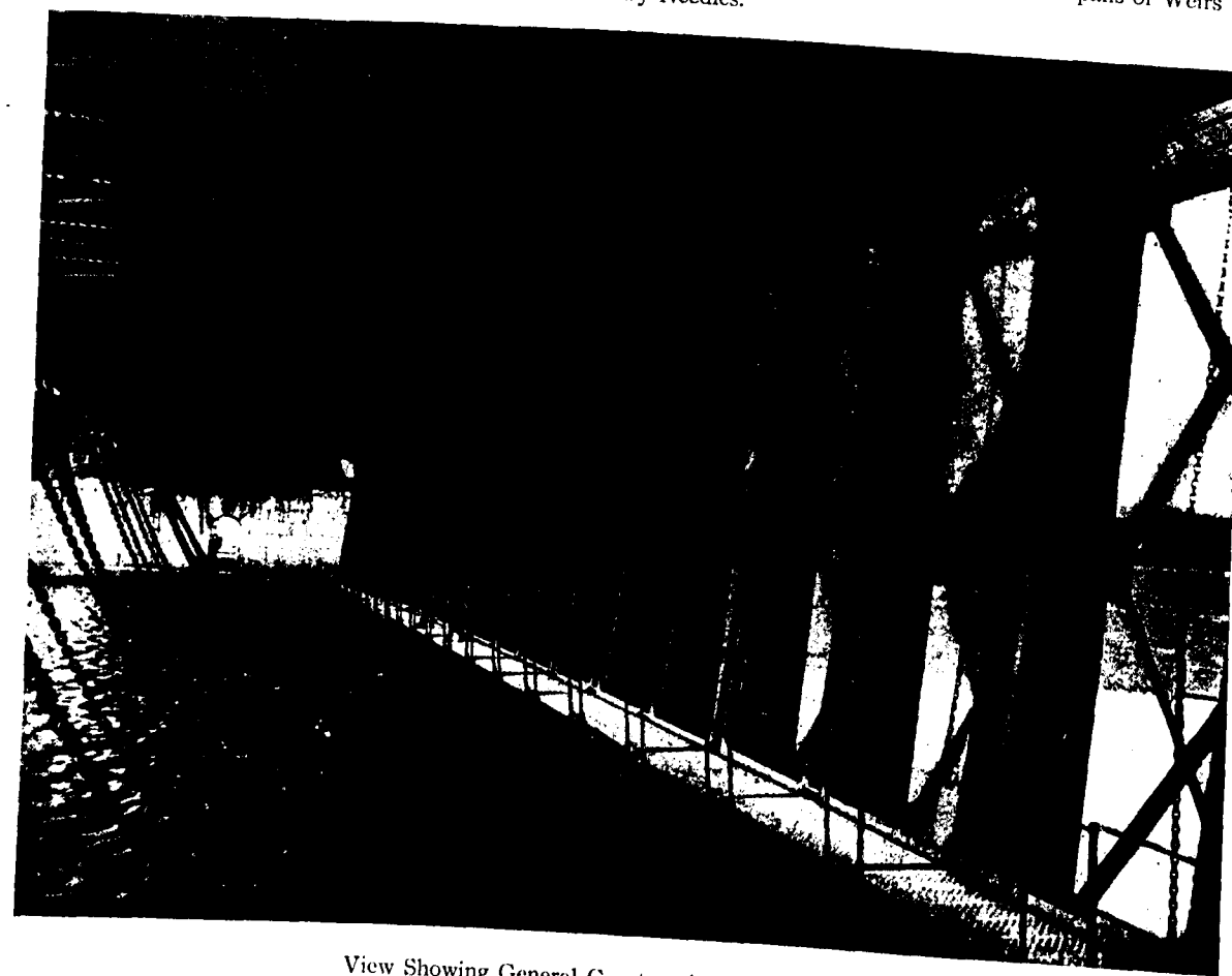
View from above Dam, Showing Dam in Position. Center Span or Pass closed by Gates, Side Spans or Weirs closed by Needles.
