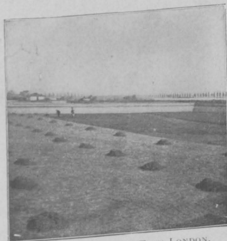
CLEANING A FILTER, EAST LONDON.
