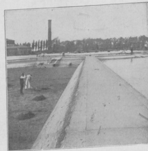
PAVED EMBANKMENT BETWEEN TWO FILTERS, EAST LONDON.
