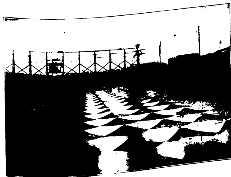
PLACING THE FLOOR OF A FILTER.
