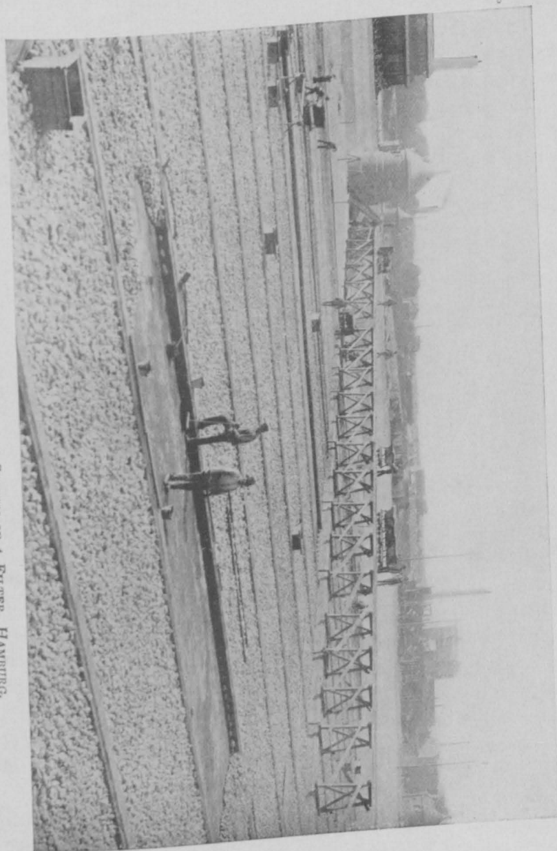
CONSTRUCTING THE UNDERDRAINAGE SYSTEM OF A FILTER, HAMBURG. [7th face page 42.]
