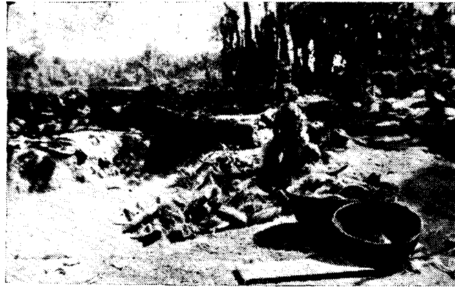
The retted husks are cleaned so as to remove dirt, etc.
