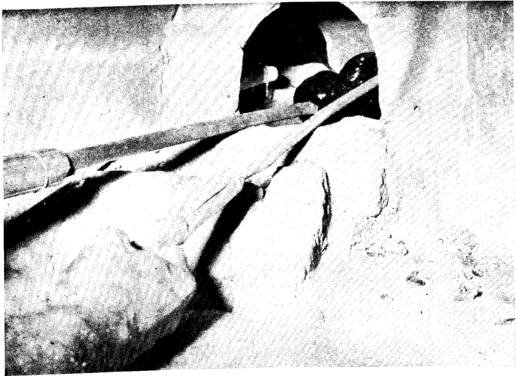
Photograph Nos. 20 and 21 Coloured sticks are prepared by mixing sheet glass and glass enamel stones. The red hot pieces of sheet glass and glass enamel stones are thoroughly mixed with the help of an Ako.li and Salukh . Note the twists given to the red hot glass mass
