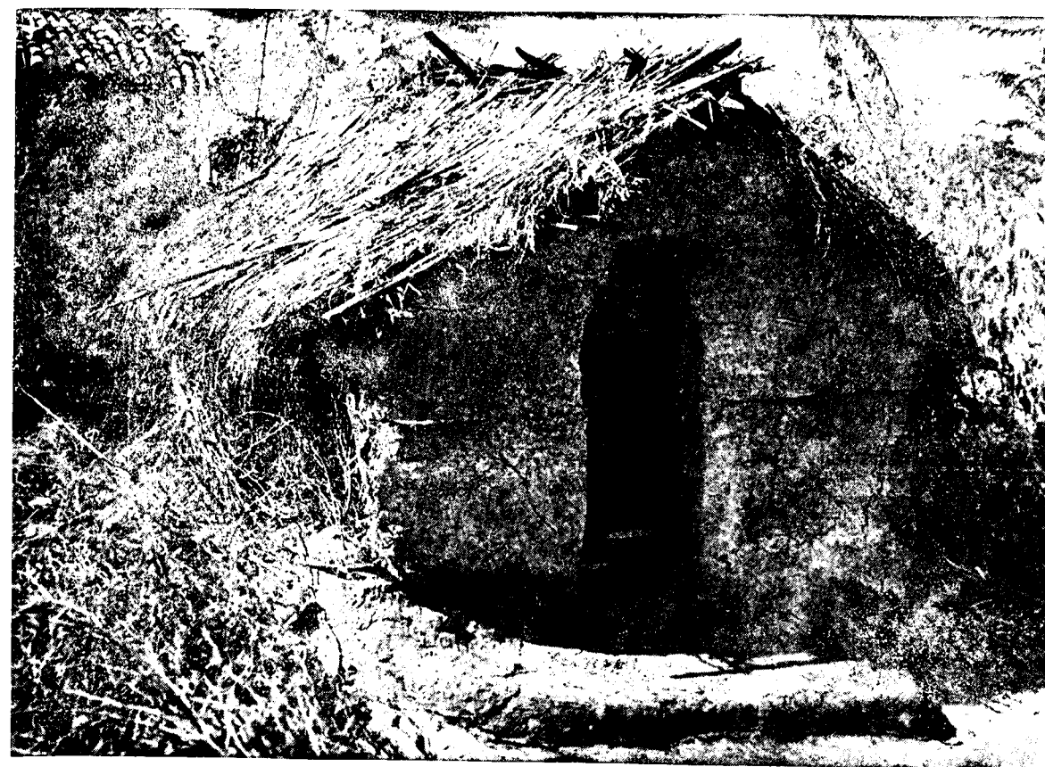
Bamboo walls plastered with clay and cow-dung covered with thatched roof
