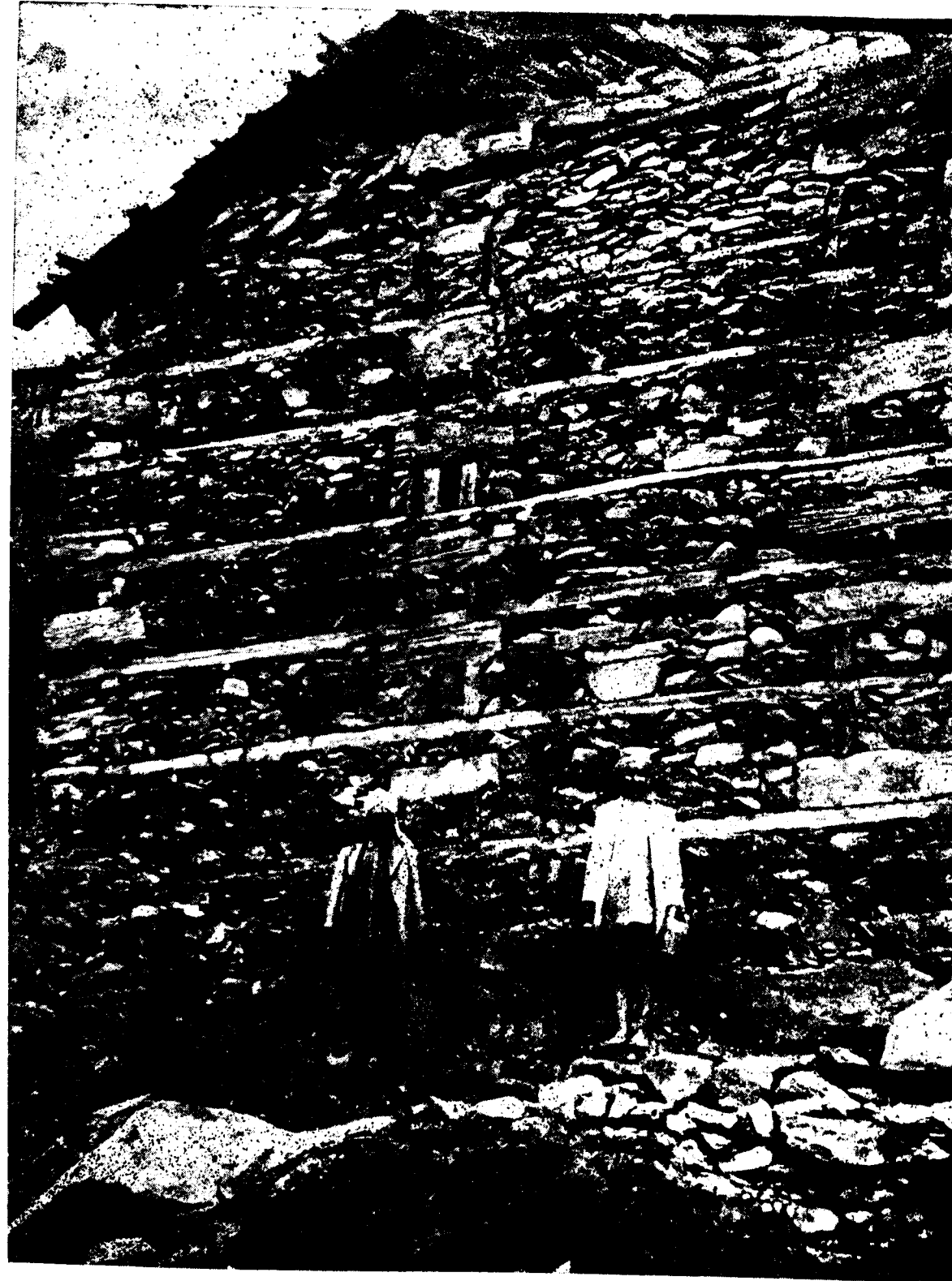
Structure of AN OLD HOUSE near Brahmaur
