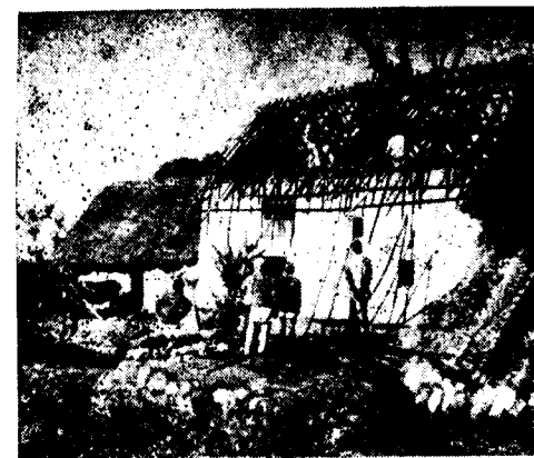
ROOF LAYING near Sarkaghat
