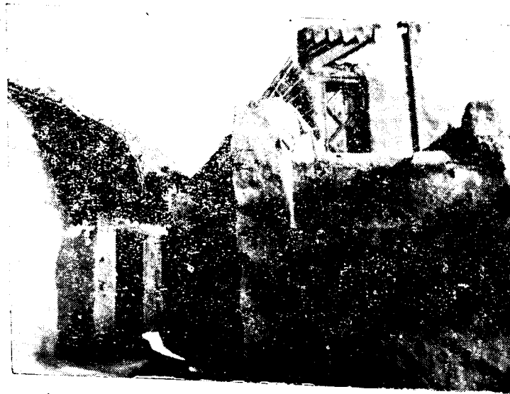
A semi-pucca house in village Barauli, Tahsil Atrauli District Aligarh (West Plain) The front walls of the house are built of burnt bricks and the remaining wall of sun-dried clay bricks. The roofs are built of mango beams covered with burnt bricks and thin mud layer. A portion has a thatch of moonj Grass
