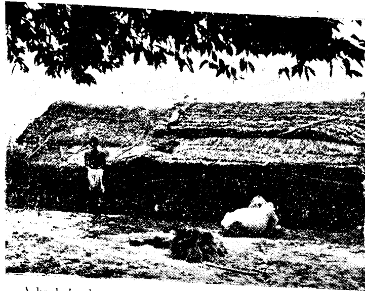
A kachcha house in village Sumbha Dih, Tahsil Ghosi, District Azamgarh (East Plain) The walls are made of reed and the roof of thatching grass
