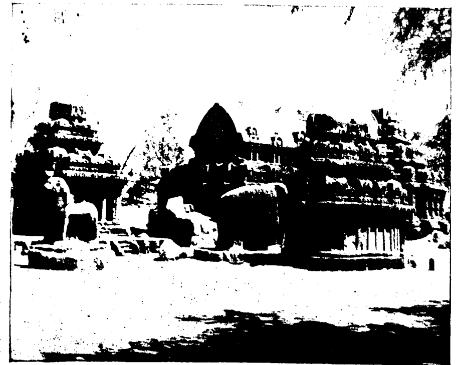
General view of the Rathas MAHABALIPURAM
