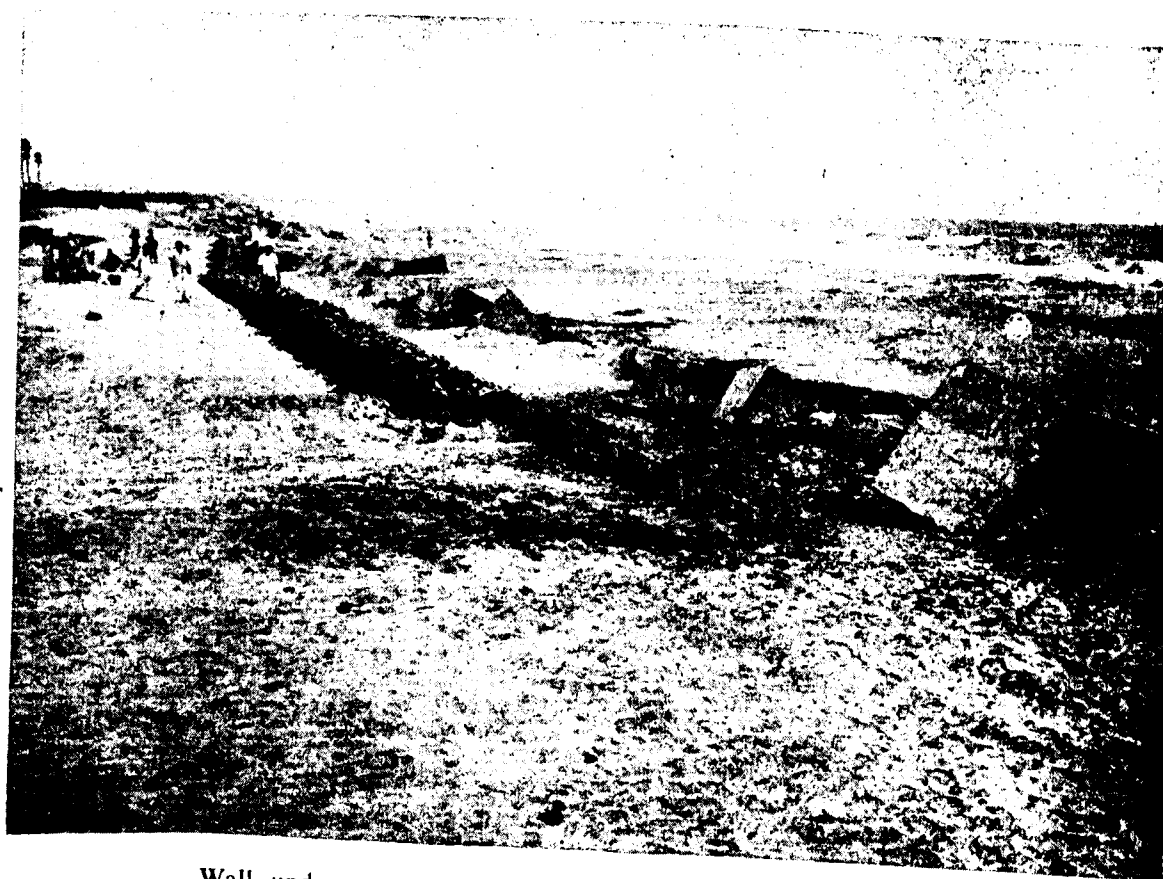
Wall under construction in Royapuram to check sea erosion
