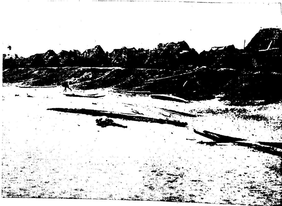
Sea erosion near a slum
