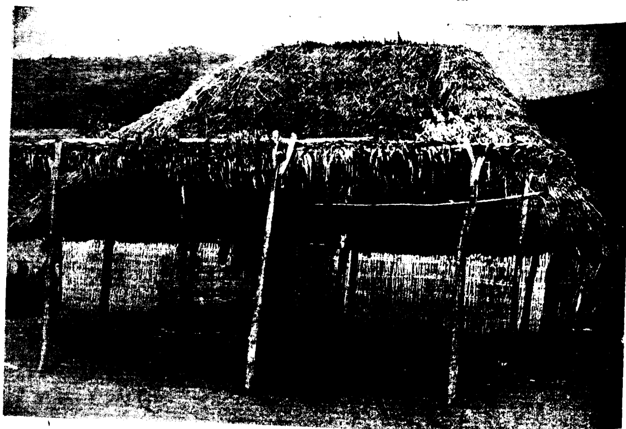
A hut of the Pachai Malayali of Pappanaickenpatti village, Salem District. The roofing is of Kanangu grass. Walls and flooring are of mud. Bamboo sticks partition the front portion into a verandah.
