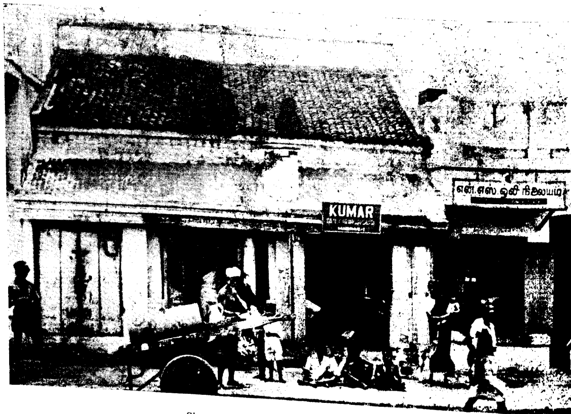
Shop - cum - dwelling in an urban area.
