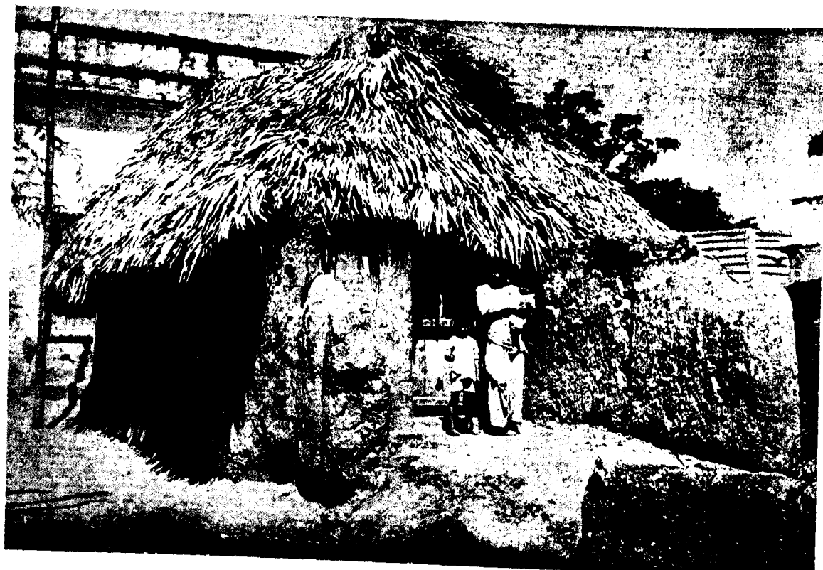
A Scheduled Caste hut in Thiruvallavayanallur village of Madurai District. Flooring is of mud and the walls are of mud too. Palmyrah thatch is used for the roof.
