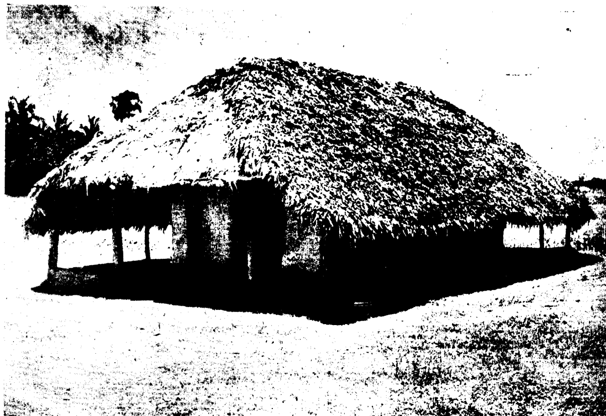
The hut of a Hindu Pallan in Vilangulam village. The walls are of mud and the roof is thatched. Two households live in this hut and so two separate entrances have been provided. It is a poor man's hut.
