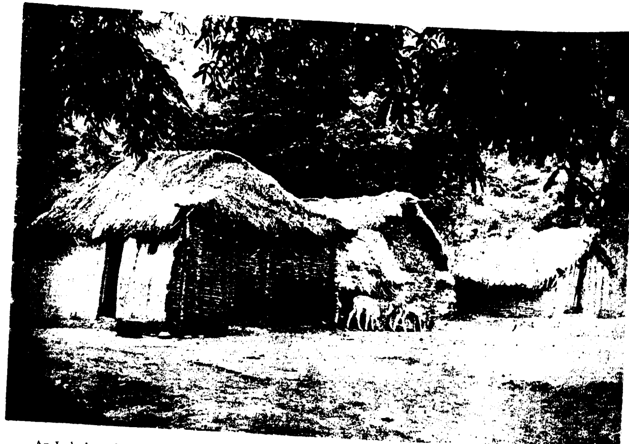
An Irula hut of Hallimoyar situated in Nilgiri District. This photograph depicts a large sized hut with two rooms where two households live in juxtaposition. Roof is of thatch and the walls are of mud.
