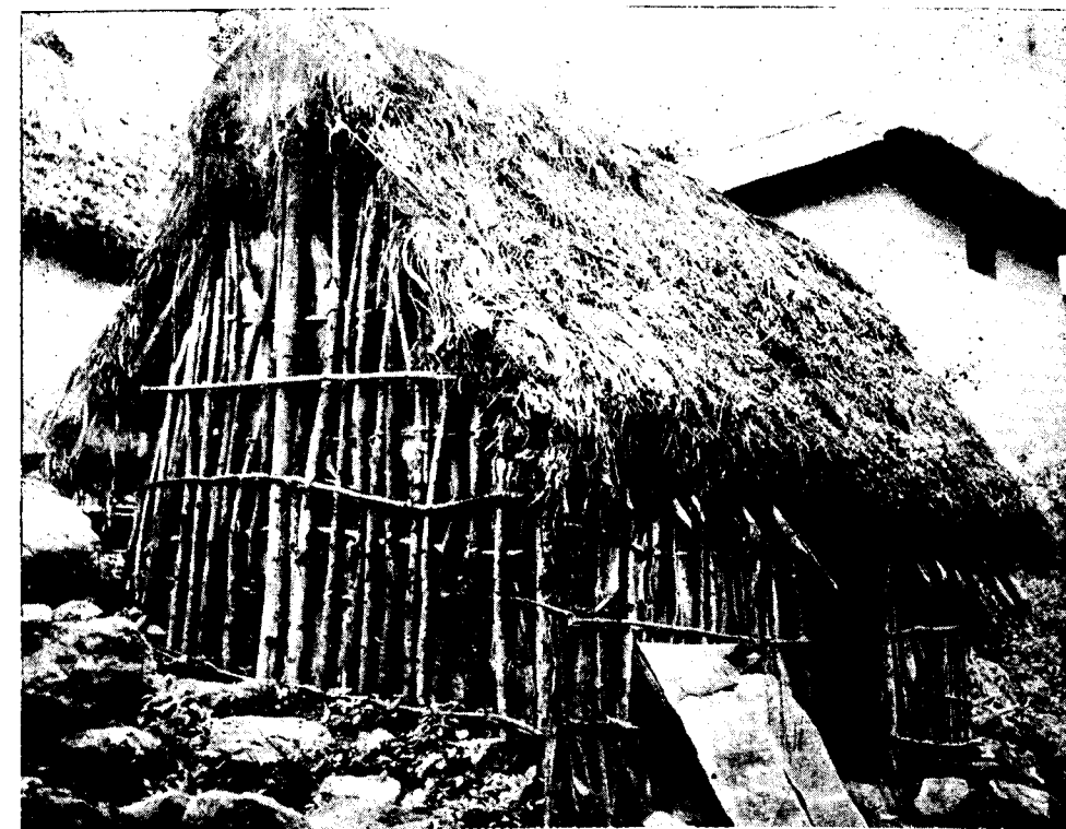
The hut of the plantation labourer and the Chakkilians. These are single roomed and the walls are of bamboo poles and banana bark. Roof is of coconut leaves and grass.
