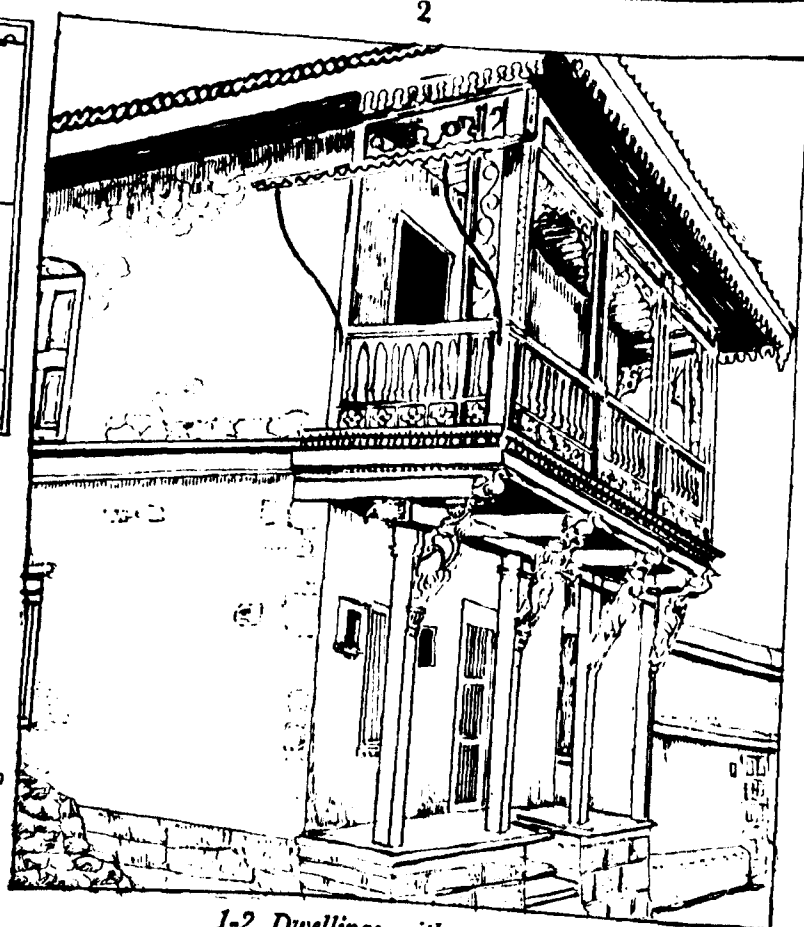
1-2 Dwellings with stone walls
