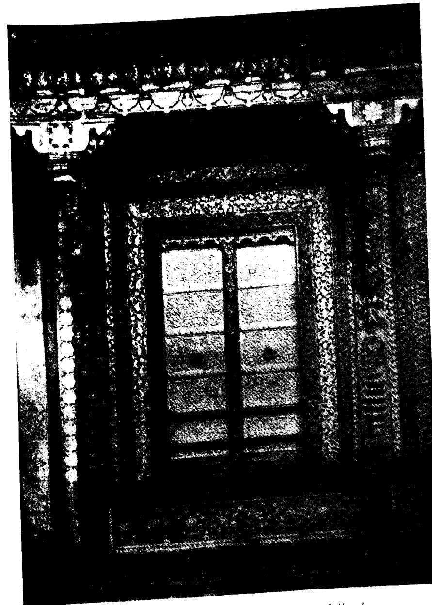
1. Carvings on window frame, doors, and lintel
