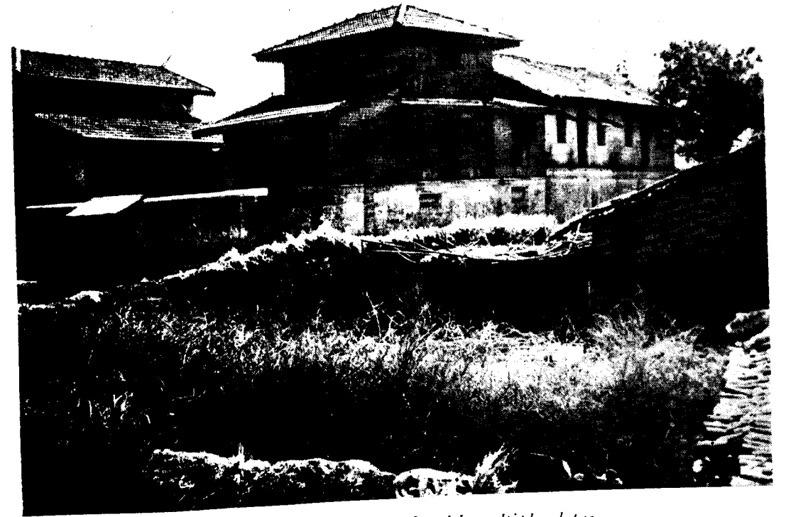
1. Brick walls and tiled roofs with multiple slopes
