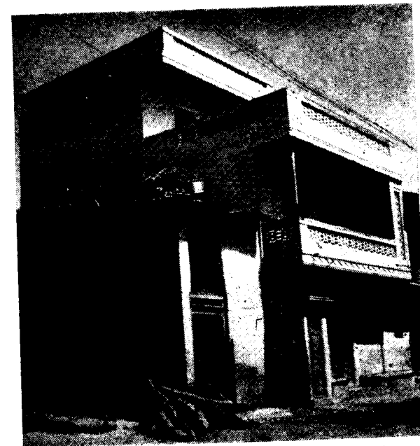
3. Brick walls plastered with cement with R. C. C. terrace
