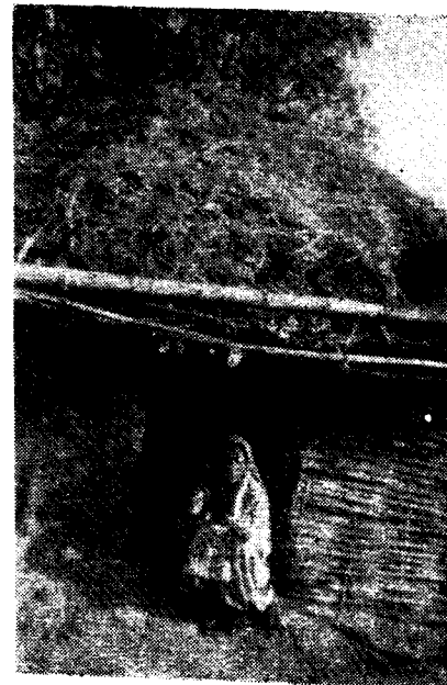
A Katkari hut in village Poshera of Mokhada taluka in Thana District Walls of reed and Roof of grass
