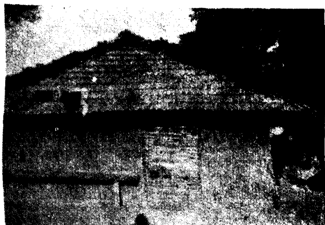
A Hut of a Ka Thakur in village Mokhada taluka Mokhada, district Thana Walls of reed ; Roof of tiles with grass for the corner joints
