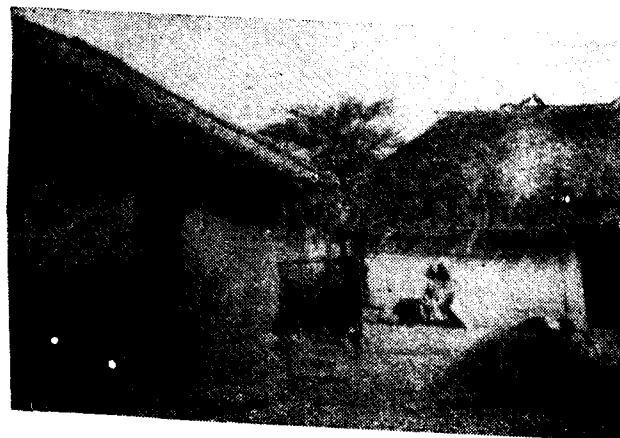
Two houses of Andh Tribe in village Daheli taluka Darwha, district Yeotmal Mark the stone plinth, walls of mud and roofs of country tiles in one and grass in the other
