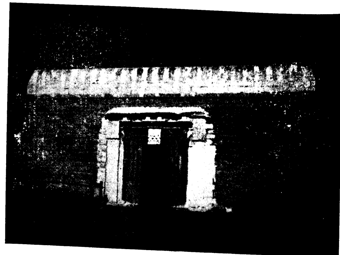
1 and 2. Stone walls with flat mud terrace.
