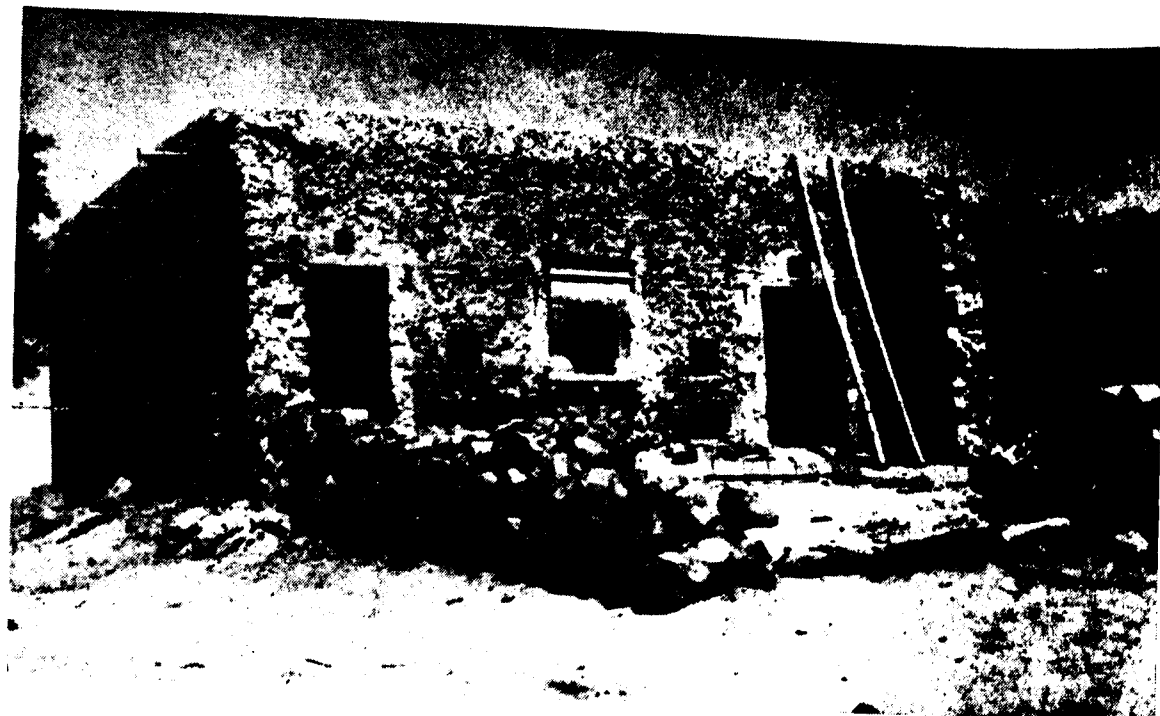
1 and 2. Stone walls with flat mud terrace.
