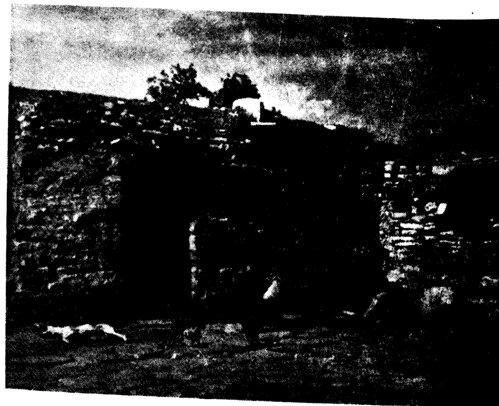
1 and 2. Stone walls with flat mud terrace.
