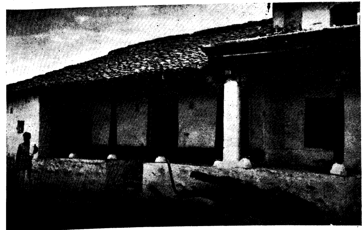
1 and 2. Mud walls with country tiled roofing.
