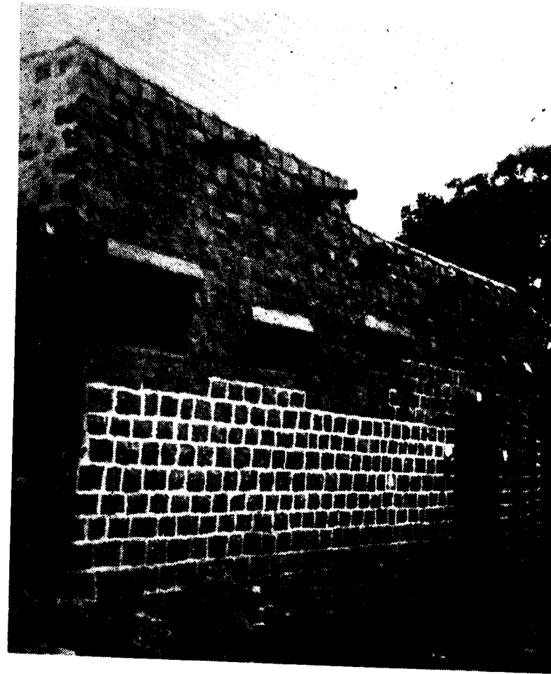
Stone walls with mud plaster covered flat mud terrace.
