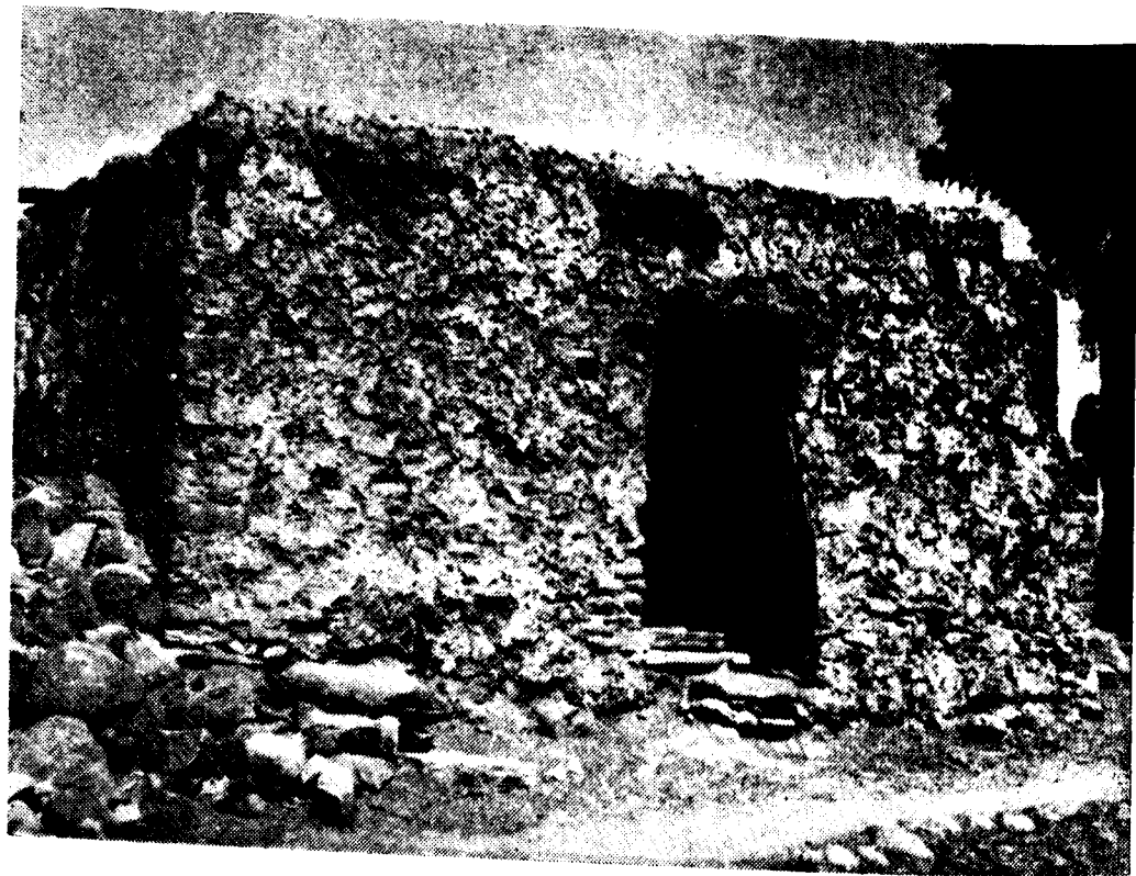
1. Stone walls with mud plaster and flat mud terrace. 2. Stone and mud walls with flat mud terrace.
