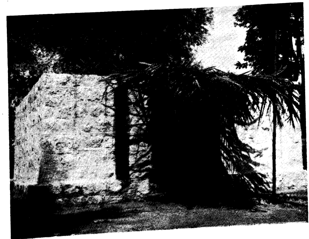
1 and 2. Stone walls with flat mud terrace.
