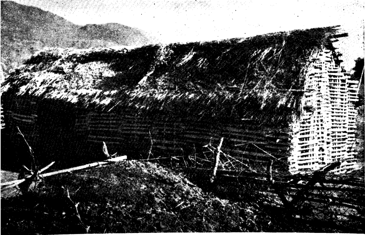
1 and 2. Bamboo reed walls and thatched roof.
