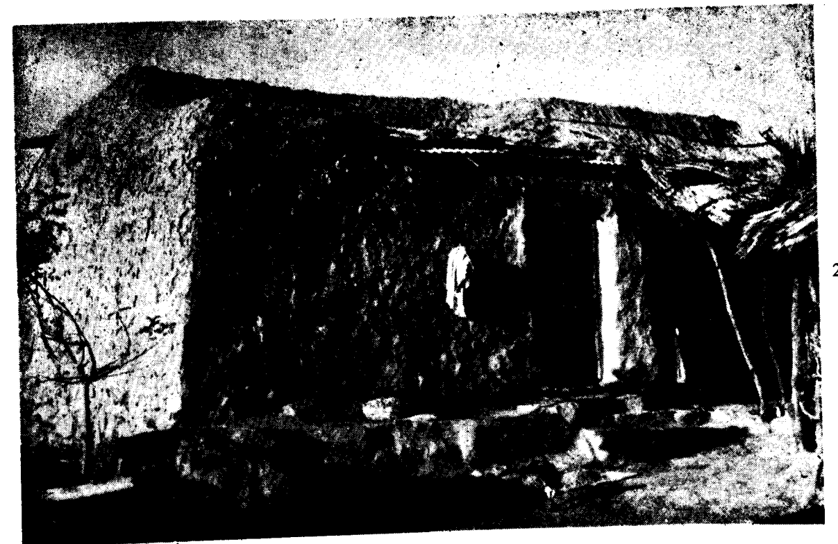
1. Mud and stone walls with flat mud terrace. 2. Stone walls with mud plaster and flat mud terrace.
