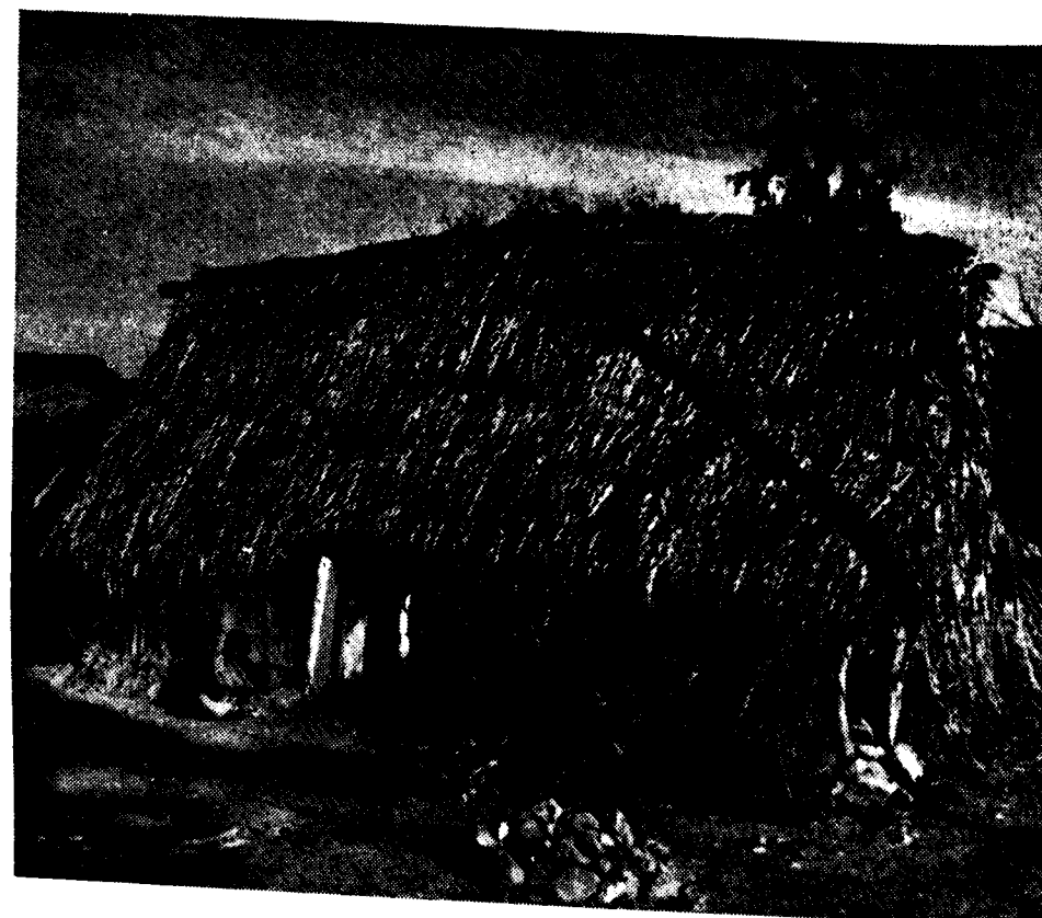
1 and 2. Walls of jowar stalk and thatched roof.
