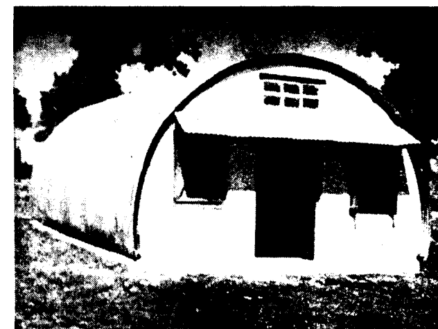
A TEMPORARY OFFICE BUILDING IN DANDAKARANYA DEVELOPMENT AREA AT UMARKOT
