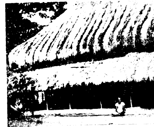
A DOUBLE-STOREYED THATCHED HOUSE OF A RICH CULTIVATOR, NORTH BALASORE ...layer of straw is thick, sometimes nearly 12 inches... (Para 98)
