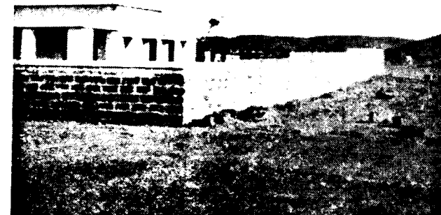
... structures like compound walls are also built of laterite stone... (Para 93)
