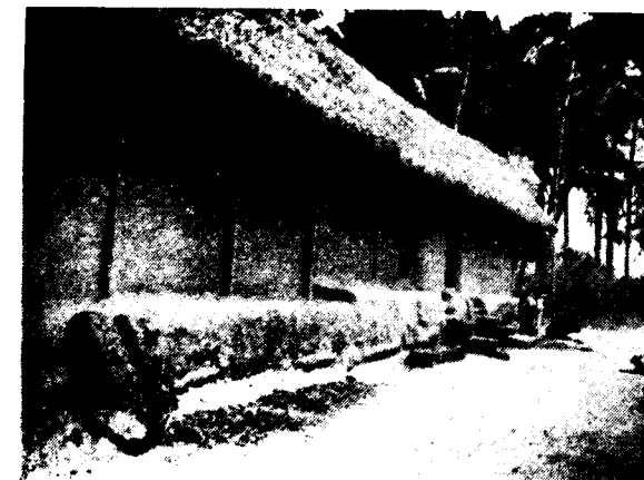
A VIEW OF BUILDING NO. 18 FROM VILLAGE STREET, PURI DISTRICT
