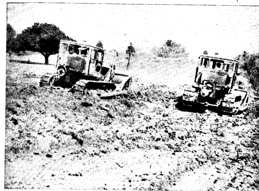
Kotaldighi given a face-lift by renovation
