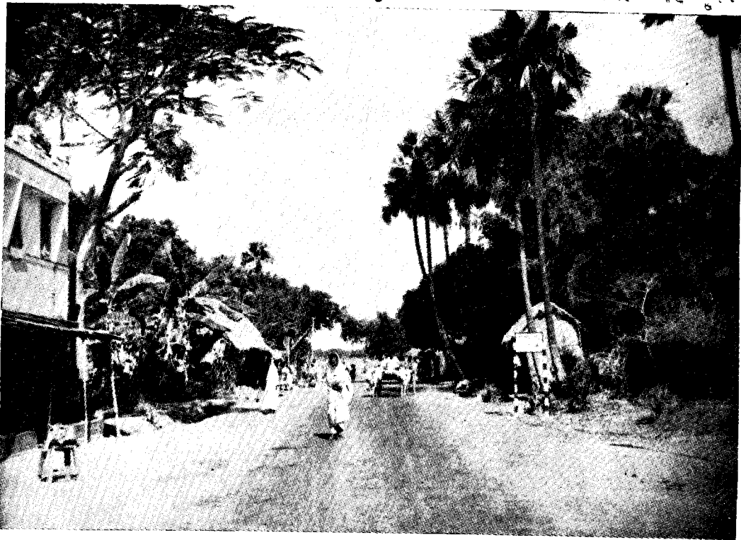
Howrah-Bishnupur metalled road—the only connecting link with the outside world
