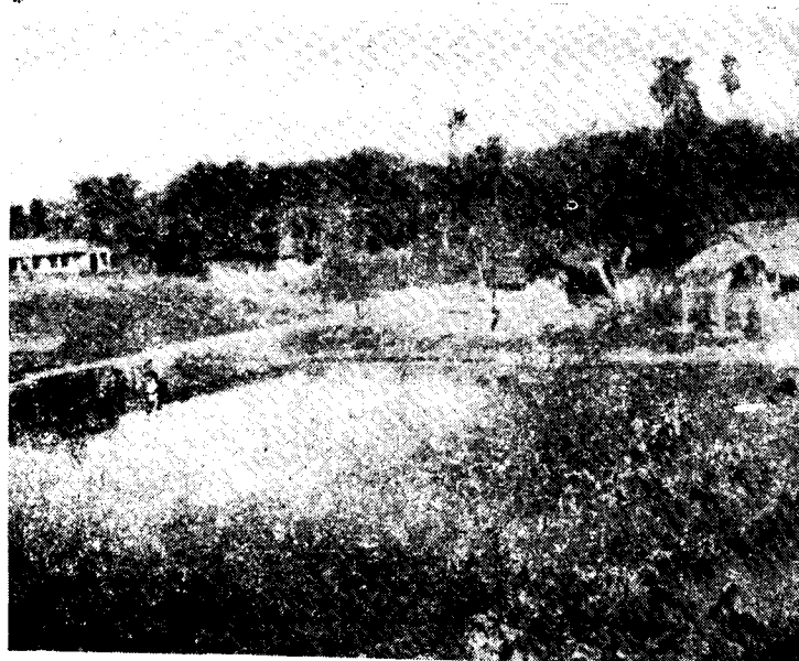
THE TANKS EXCAVATED BY THE RAILWAYS
