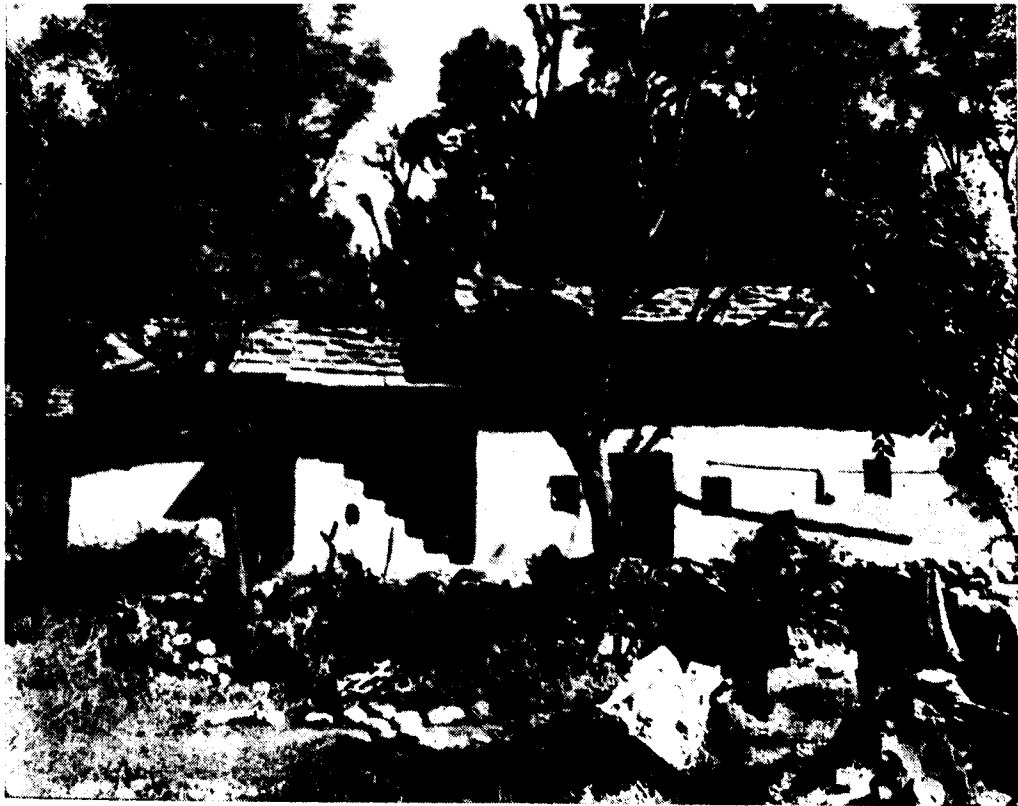
A house in village Chetru (Kangra District)—hill region with heavy rains. Note the sloping slate roofs projecting on the walls. The house belongs to a Rajput with a substantial agricultural holding.
