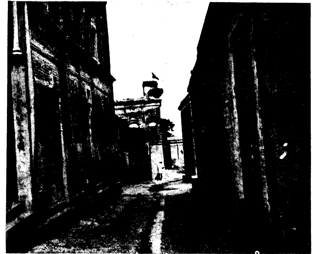
A street in Tehang, a prosperous village in Jullundur District. Note the paved street with an open drain in the centre.
