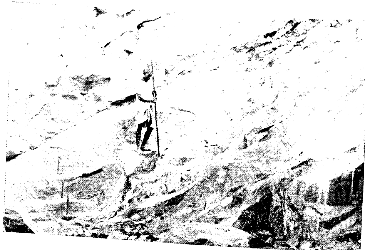
16. Drilling a quarry before blasting.
