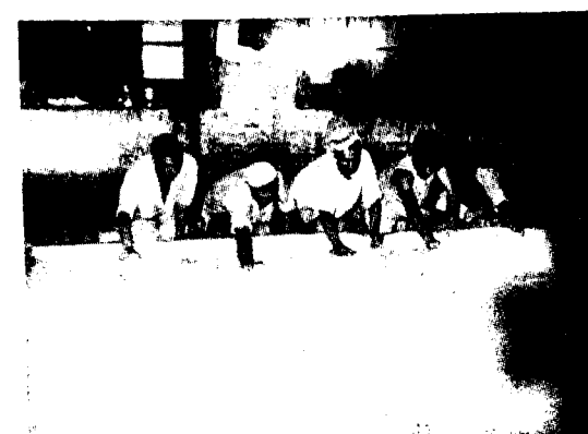
The Namdah is rubbed with soap while still on the mat and is afterwards transferred to a specialist for washing
