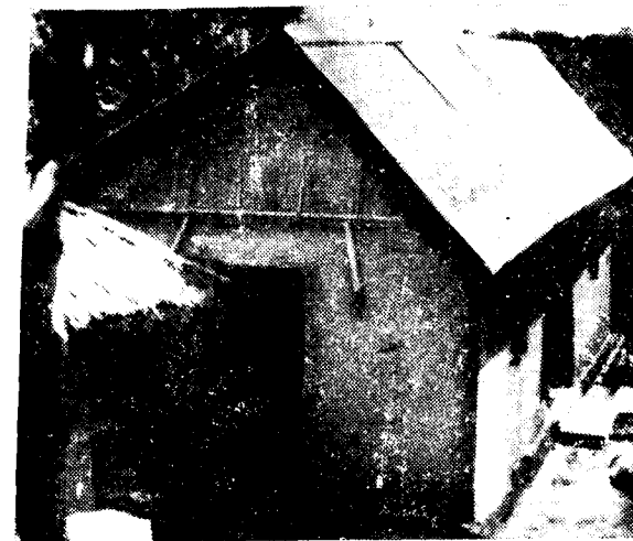
No. 13. SHOWING WALLS OF MUD AND ROOFS (TWO) OF C. I. SHEET.
