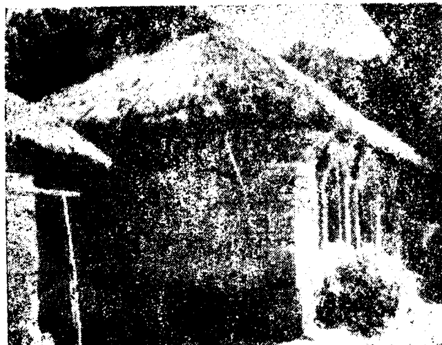
No. 7. SHOWING WALLS OF UNBURNT BRICKS AND ROOFS (TWO) OF SAN-GRASS.
