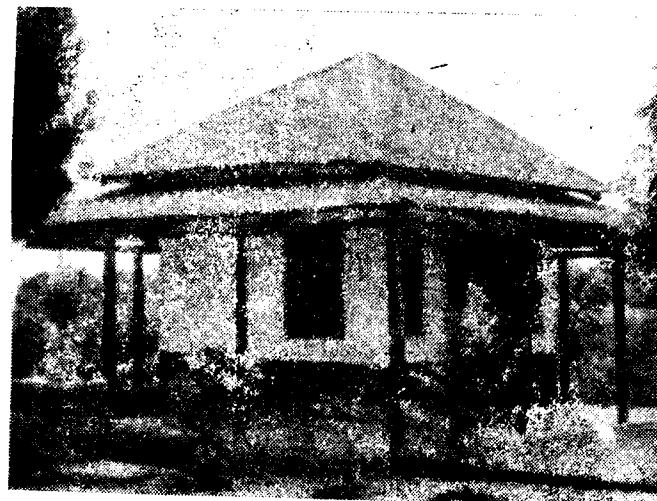
No. 18. SHOWING PUCCA WALL OF BURNT BRICKS AND ROOF WITH HIPPED RIDGES.
