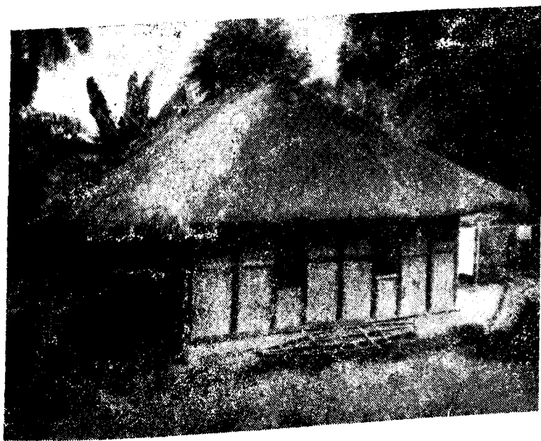
No. 2. SHOWING WALLS OF BAMBOO TARJA AND ROOFS (FOUR) OF SAN-GRASS.
