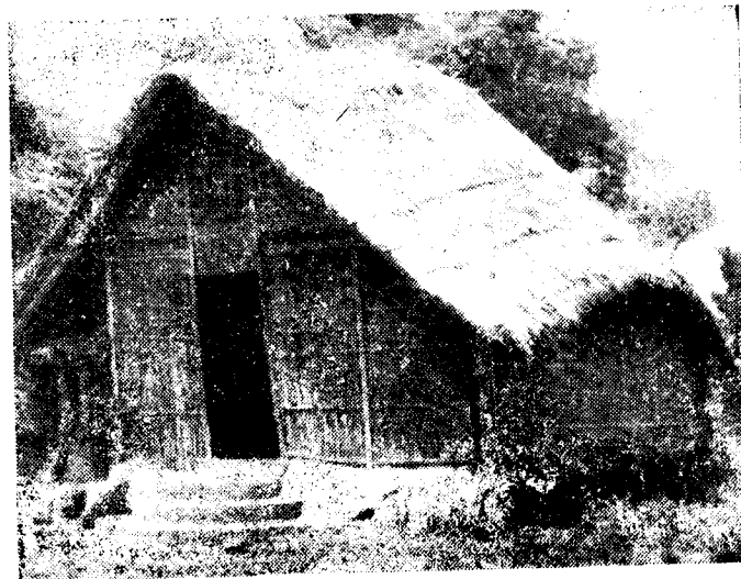
No. 3. SHOWING WALLS OF REEDS AND HORIZONTAL SPLIT BAMBOO BATTENS WITH OR WITHOUT PLASTERING OF MUD AND ROOF (TWO) OF SAN-GRASS.
