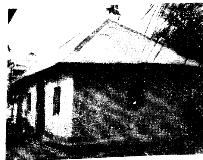
No. 14. SHOWING WALLS OF MUD AND ROOFS (FOUR) OF C. I. SHEET.
