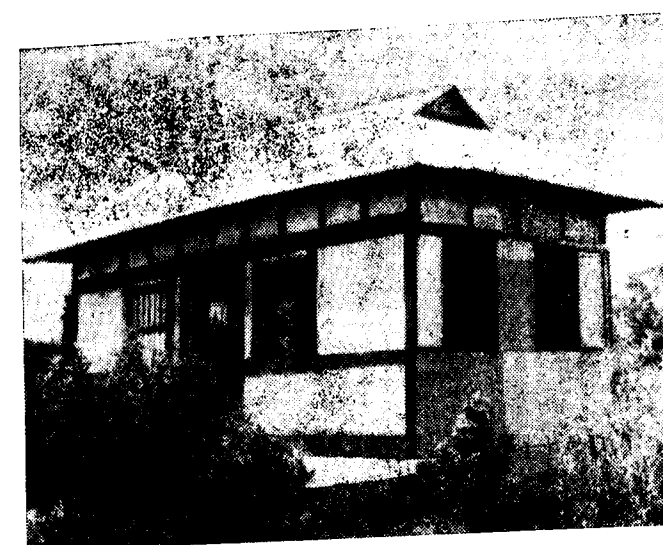
No. 17. SHOWING WALLS OF C. I. SHEET AND ROOFS (FOUR) OF C.I. SHEET IN GABLE TYPE.
