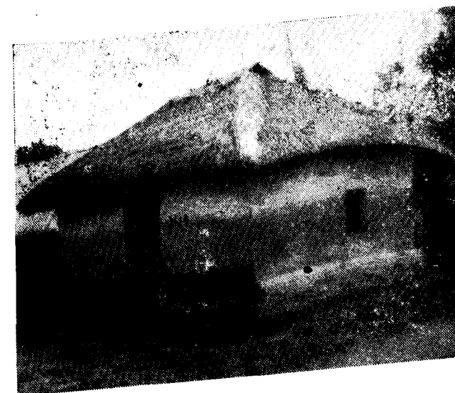
No. 6. SHOWING WALLS OF MUD AND ROOFS (FOUR) OF SAN-GRASS.
