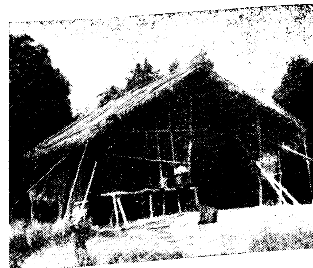
No. 9. ANOTHER "TONG" HOUSE IN TRIBAL AREA—WALLS OF SIMPLE BAMBOO TARJA AND ROOFS (TWO) OF SAN-GRASS. FLOOR OF BAMBOO 3' ABOVE THE GROUND LEVEL.
