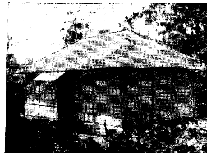
No. 20. SHOWING WALL OF BAMBOO TARJA AND ROOFS (FOUR) OF OTHER METAL SHEET.
