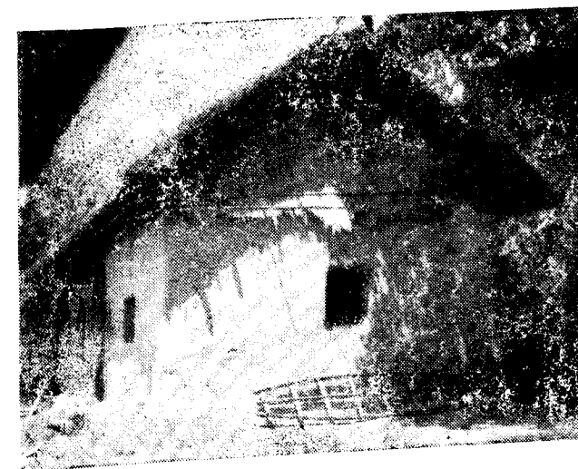
No. 5. SHOWING WALLS OF MUD AND ROOFS (TWO) OF SAN-GRASS.
