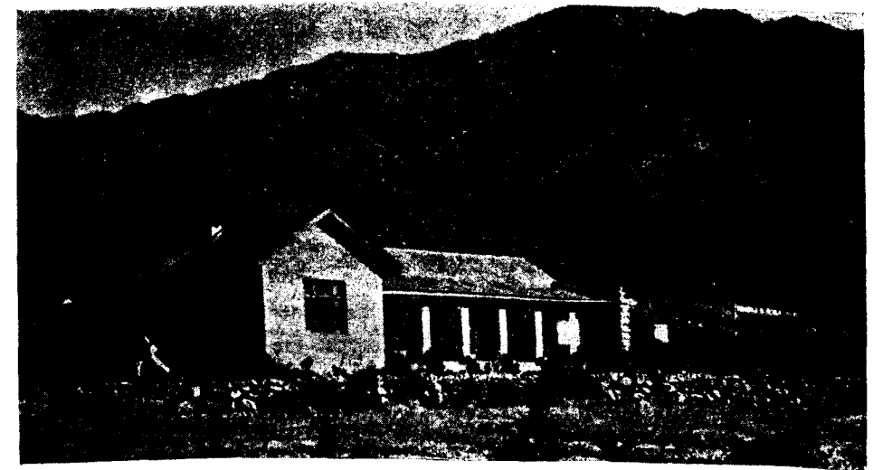
The village high school building
