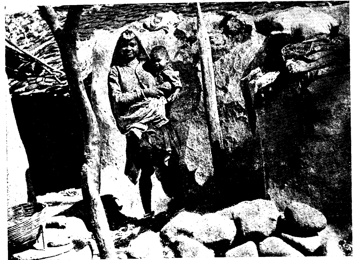
Repairs to a house
