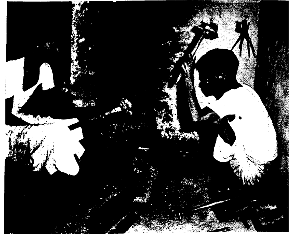
Sl. No. 21 (Photo plate 14758) Hammering the thori (lower part of a betel-nut cracker).
